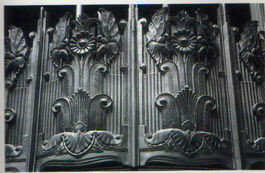
1 Original blueprints showing elevations (Opposite) 2-4 Architectural details fill the building 5 Lift lobby 6 American International Building in the New York skyline 7 View of the American International Building Photography: courtesy American International Realty Corp.
