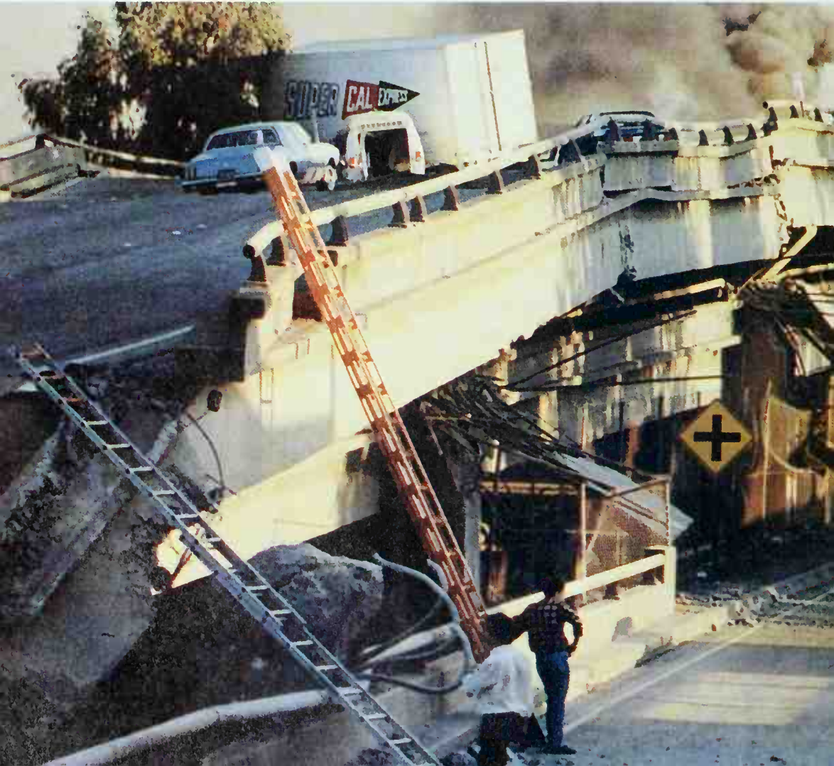
earthquake damage, San Francisco
