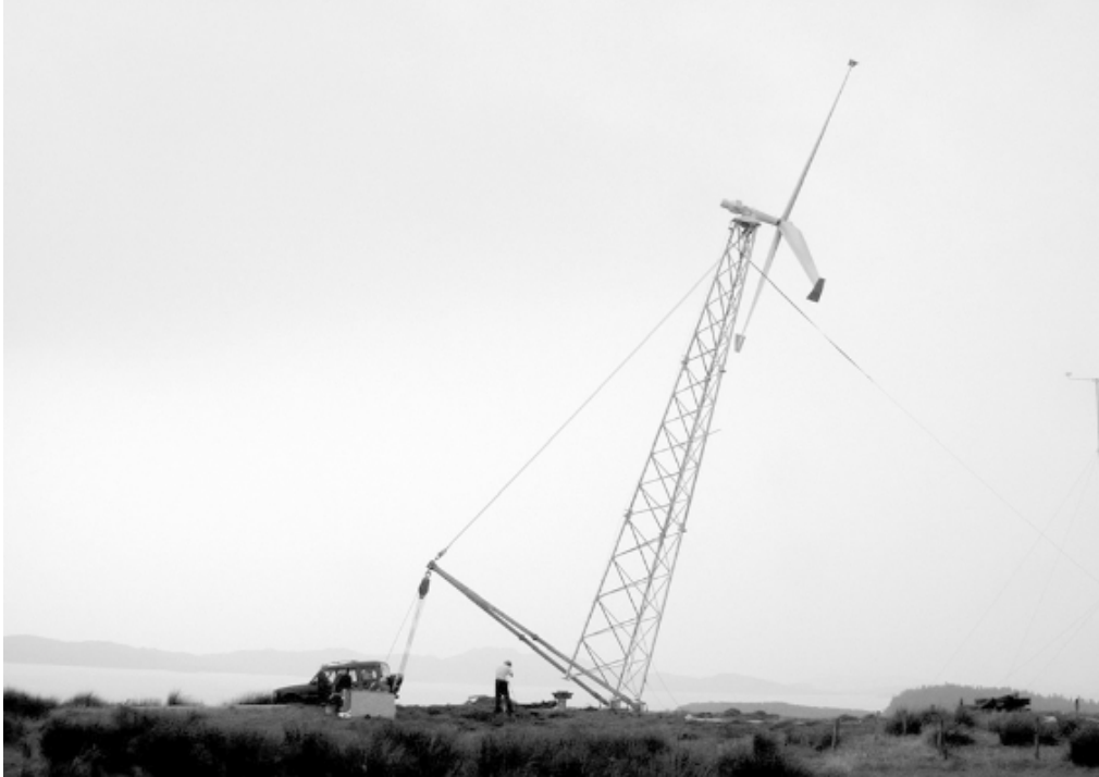
Figure 9.27 Winch erection of a 50 kW wind turbine. Winch loading is highest at the start of the lift when the weight moment is greatest; once near the vertical, the winch load reduces almost to zero: the back stay seen on the right will shortly take up the load. (Photo courtesy Paul Pynn)
