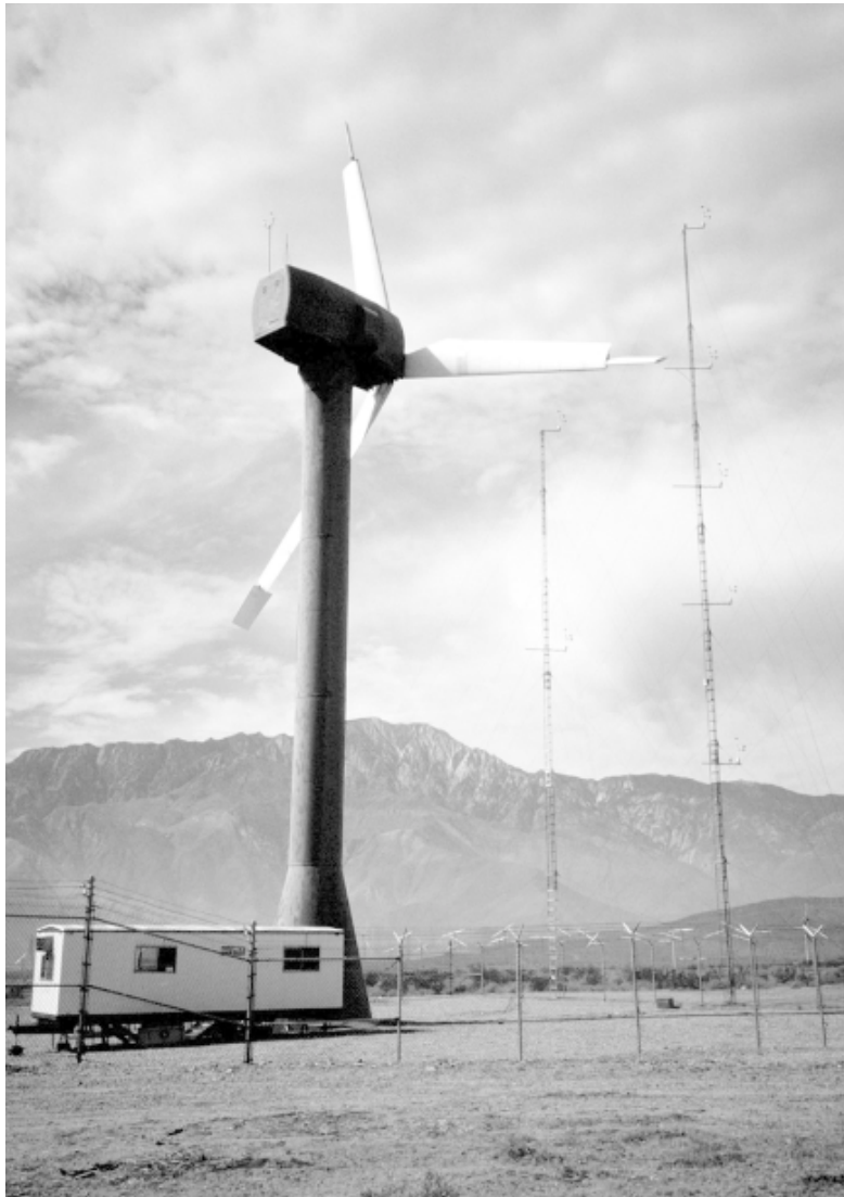
Figure 7.24 The Howden HWP26 wind turbine at the SCE test site in Palm Springs, 1986.
