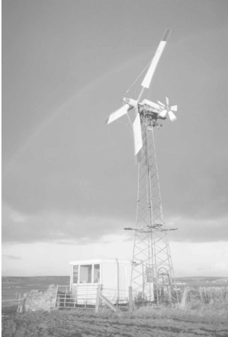
Figure 1.4 A Danish classic. Christian Riisager's 1975 design was the first series-produced wind turbine, rated at 22 kW and manufactured with off-the-shelf components. The example shown was installed on South Ronaldsay on Orkney in 1982. Note the fantail yaw drive, echoing traditional windmill designs.
