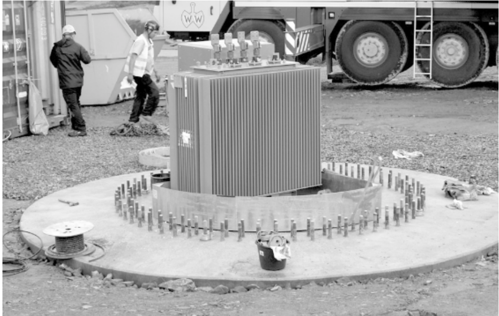
Figure 9.29 Transformer for an 800 kW wind turbine. The lowest tower section will be lowered into place over the top of the transformer, with the control cabinets installed in a floor immediately above.
