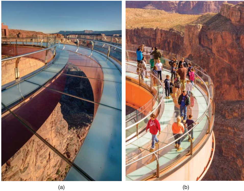
Figure 5.30 Grand Canyon Skywalk imaging. (a) Laminated glass floor. Source: Photo by Aerographics. Reproduced with permission from Grand Canyon Resort Corp. (b) Access with special shoes only. Source: Photo by Madison Kirkman. Photography reproduced with permission from Grand Canyon Resort Corp.
