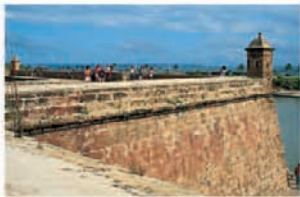
Section of Palma's city walls
