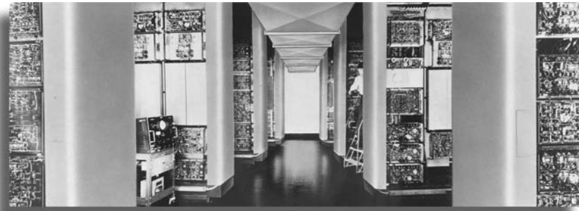
Interior of the Barta Building with the Whirlwind computer, 1951. (Courtesy of MITRE Corporation.)
