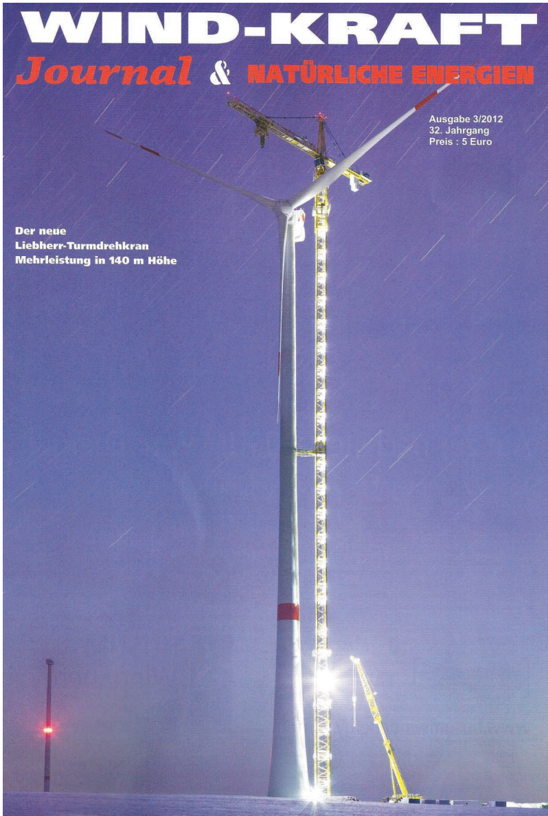
Figure 7.3 The elegant 140 m-high tower of a modern wind turbine with its assembly crane.
