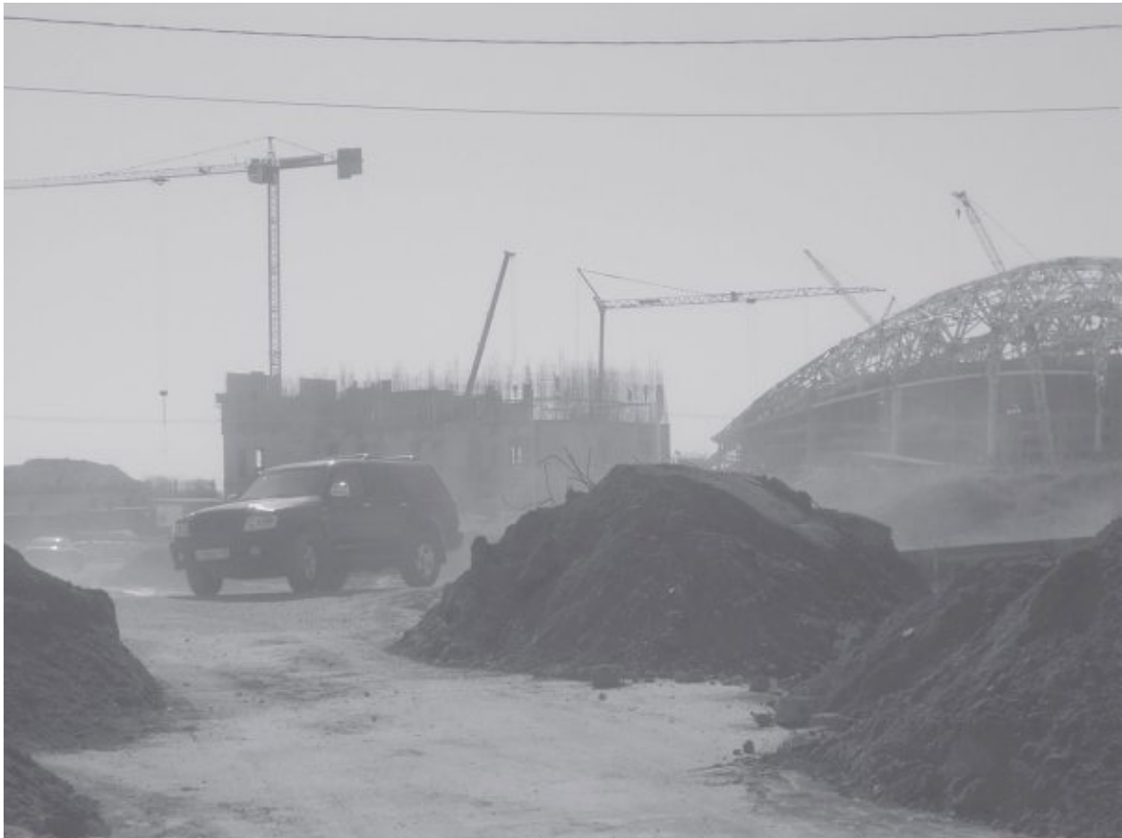
My favorite picture! Terminator style. Construction of the laboratory, September 2012.
