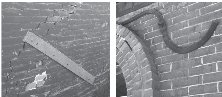
Steel masonry reinforcements.
