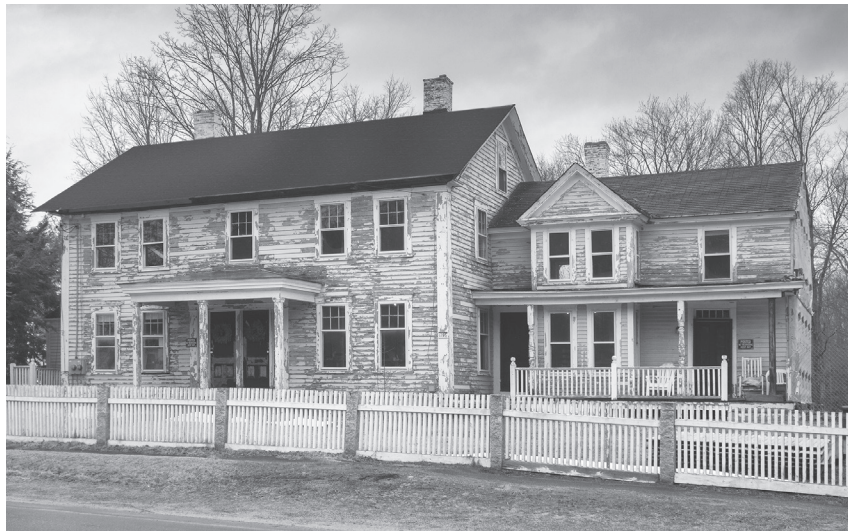
Classic balloon frame–constructed house. Note that all the doors and windows line up vertically and are the same width.
