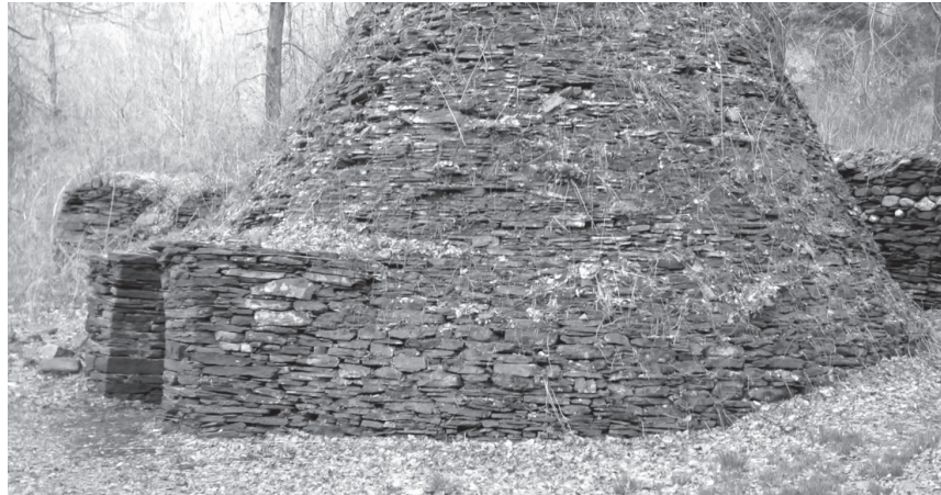
This beehive kiln played a key role in refining metals used in Civil War weaponry.
