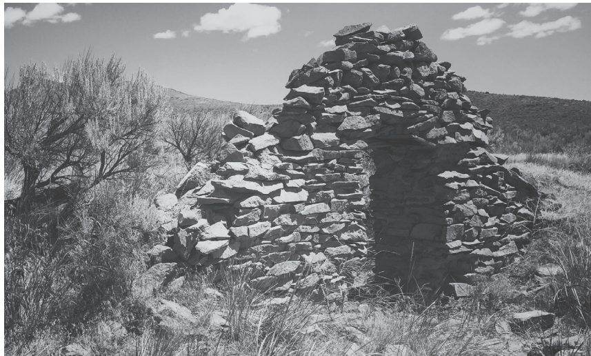
An example of dry-stacked native stone in southeast Oregon. This was the entrance to the cold storage area in the back of a late-1800s store.
