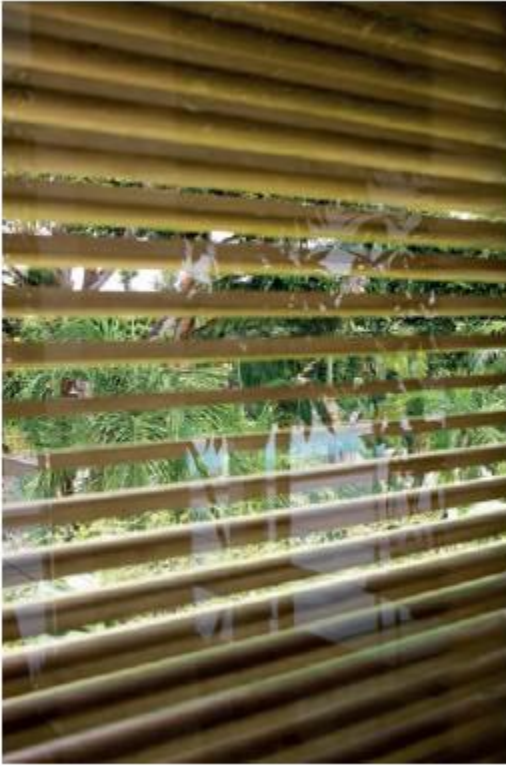
A detail of the screen that filters light into the living/dining pavilion.
