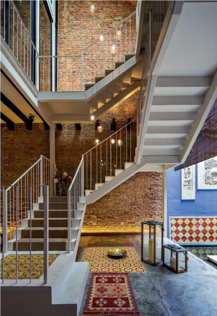
A new steel stairway connects the ground and upper floors of the original house.
