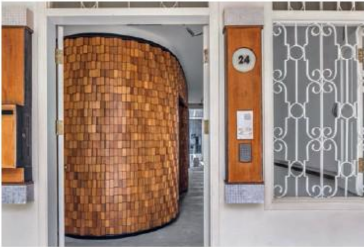
The curved textured timber wall, which contains a ground floor apartment in No. 24 Crane Road.
