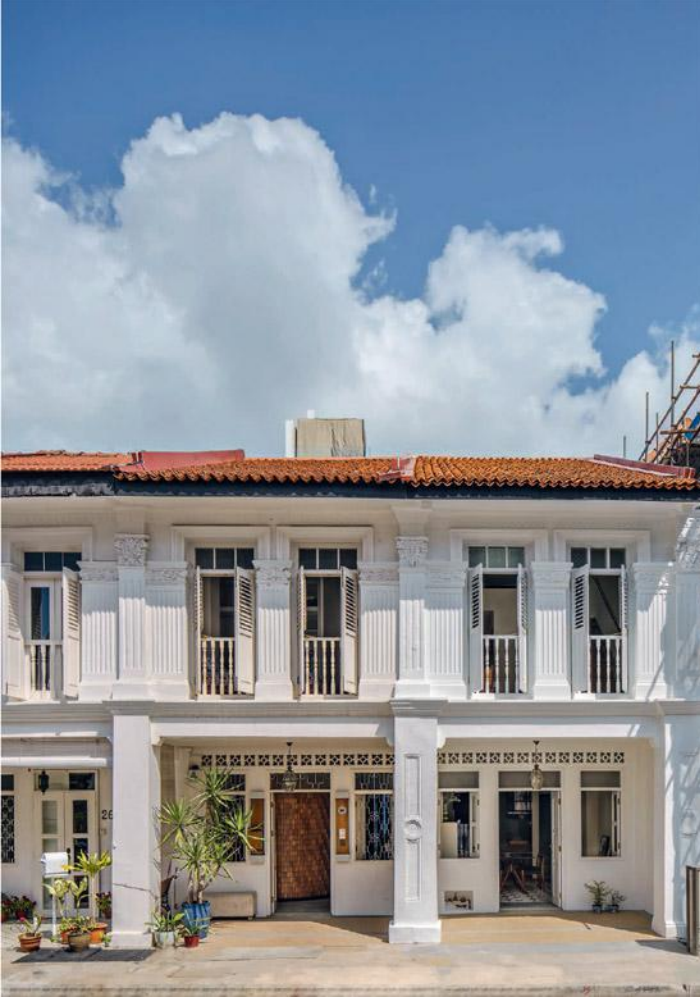
The restored street façades of the two, now connected, shophouses.
