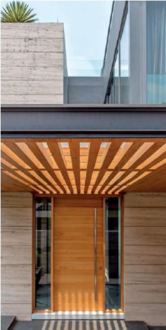
The timber-screened porte cochère, with the entry door placed between the two pavilions of the house.
