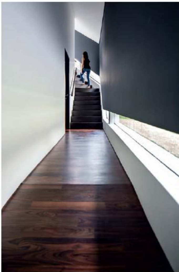
An elegant timber stairway at the rear of the bedroom pavilion links each level.
