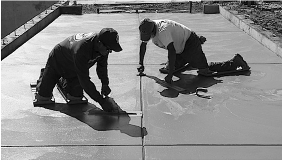
Figure 10.8 Control Joints in a Concrete Slab
