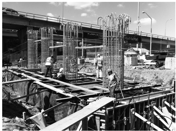
Figure 10.38 Circular Column Reinforcing
