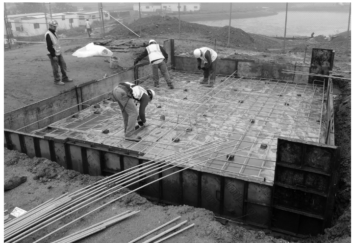
Figure 10.7 Placing Steel Reinforcing in a Concrete Slab
