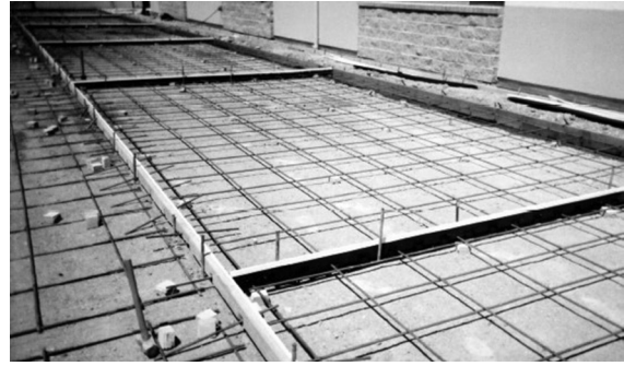
Figure 10.9 Expansion Joints in a Concrete Slab
