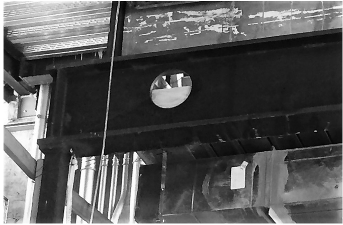
Figure 4.10 Penetration in Web of a Beam
