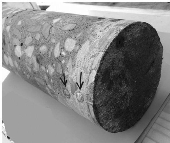
Figure 10.3 Concrete Cylinder Core
