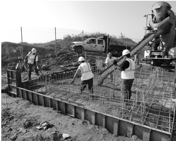
Figure 10.4 Pouring Concrete
