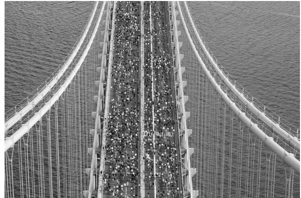
Figure 2.5 Live Load—runners on a bridge
