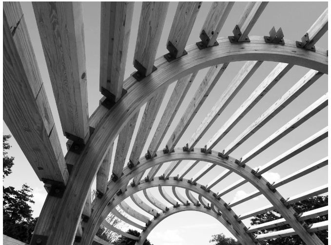
Figure 7.11 An Engineered Glulam Structure
