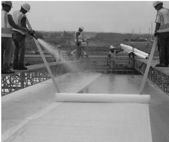
Figure 10.5 Curing of Concrete
