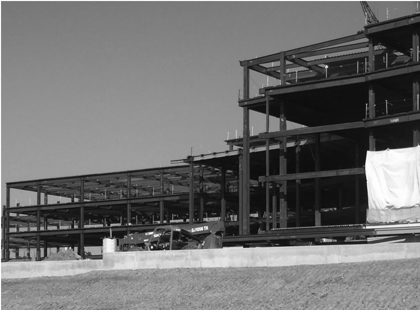
Figure 5.1 A Steel Frame Building
