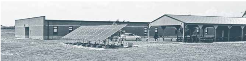
Figure 1.3. This solar array was installed at the Owensville Middle School in Owensville, Missouri, by the author and his business partner, Tom Bruns, and numerous hard-working students. The array is small for a school of this size, which uses almost 1,000 kilowatt-hours per day; the array only provides about 12 days' worth of electricity to the school. The array is also used for science and math education. Credit: Dan Chiras.
