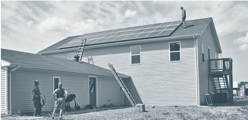
Figure 8.19. Standoff Mount. Standoff mounts allow modules to be mounted parallel to the roof, permitting PV systems to blend in better, a feature that is desirable to homeowners, business owners, neighbors, and passersby. This array was installed by me, my business partner, and a former student on Victor Pipe and Steel in Winfield, Missouri. Credit: Dan Chiras.
