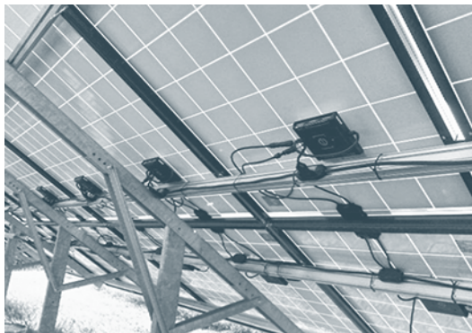
Figure 5.4. Microinverter on an Array. Microinverters like the one shown here are mounted either on the module frames or the rack system in close proximity to PV modules. They convert the DC electricity into 240 V AC electricity.
