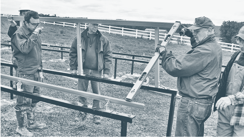
Figure 8.6. Telescoping Legs. Telescoping legs, like the ones on TEI's first solar array in 2009, allow for infinite adjustability within a range dictated by the length of the two aluminum pieces, as shown here. Here, students and a veteran installer (Bob Solger) who helped teach this workshop check the angle and distance from the front to the back rail. Credit: Dan Chiras.
