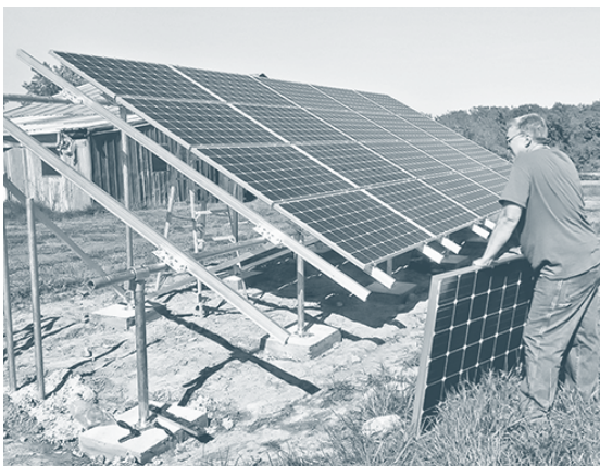
Figure 3.4. Monocrystalline Module. Monocrystalline solar cells are sliced from a long cylindrical ingot of silicon doped with boron. You can identify the type of solar cell by its distinct shape, as described in the text. Credit: Dan Chiras.
