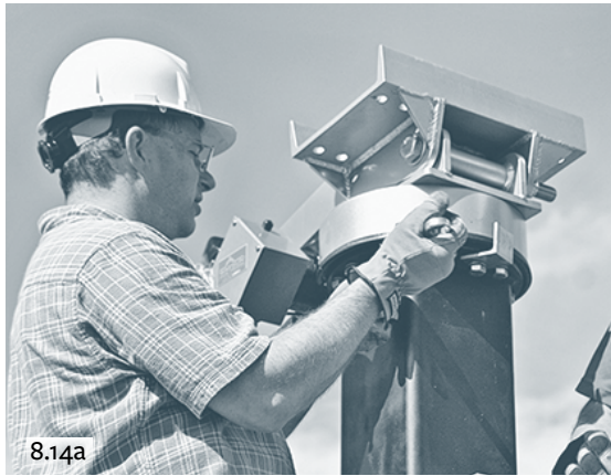
Figure 8.14. (a) Motor That Adjusts Azimuth Angle. This motor sits atop the pole and adjusts the azimuth angle of the array to track the Sun on its east-to-west path across the sky.
