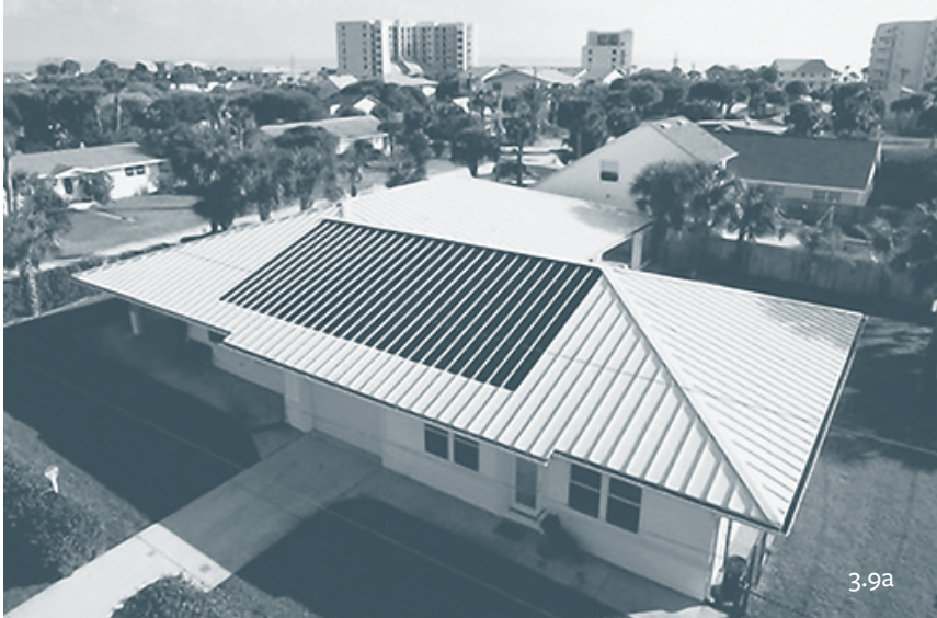
Figure 3.9. (a) PV laminate is applied directly to a standing seam metal roof as shown here. Credit: National Renewable Energy Laboratory. (b) Solar Used for Standing Seam Metal Roof. This photo shows solar laminate, or PVL, from Uni-Solar made from amorphous silicon. This product can be applied on new or existing standing seam metal roofs. Credit: Energy Conversion Devices/Uni-Solar.
