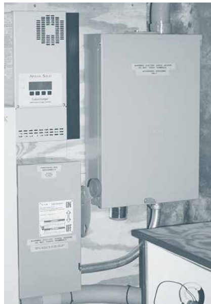
Figure 7.15. Charge Controller. Charge controllers like the one top left from Apollo Solar regulate the flow of electricity to the batteries in off-grid and grid-connected systems with battery backup. Some charge controllers contain maximum power point tracking circuitry to optimize array output and other features as well, like digital meters that display data on volts, amps, and electricity stored in battery banks.
