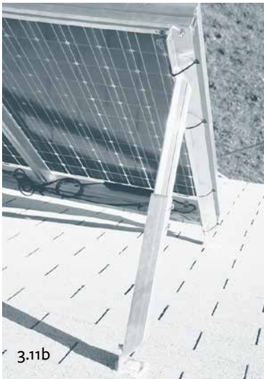
Figure 3.11. (a) Bifacial modules like those installed at the Midwest Renewable Energy Association harvest solar energy off both sides of the modules, although the front side shown here is by far the most productive source of electricity. (b) Sunlight reflecting off the light-colored roofing illuminates the back of the array, boosting its output.
