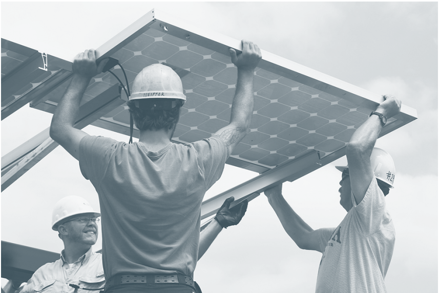
Figure 8.9. Module Being Inserted in Pole-Mount. Workers carefully slide PV modules into place on this dual-axis tracker at a Midwest Renewable Energy Association workshop in Minnesota. Credit: Dan Chiras.
