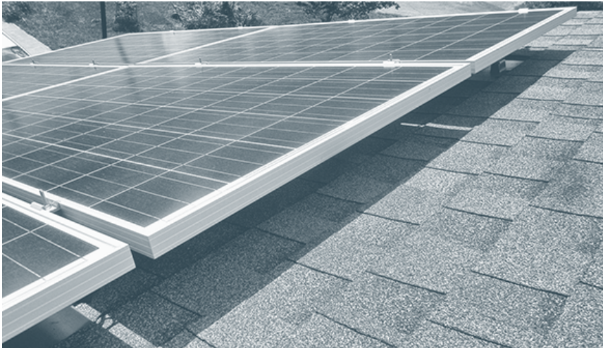
Figure 8.22. Standoff Mount. Standoff mounts like the one shown here allow modules to blend with the architecture, making them more aesthetically appealing to many individuals. Credit: Dan Chiras.
