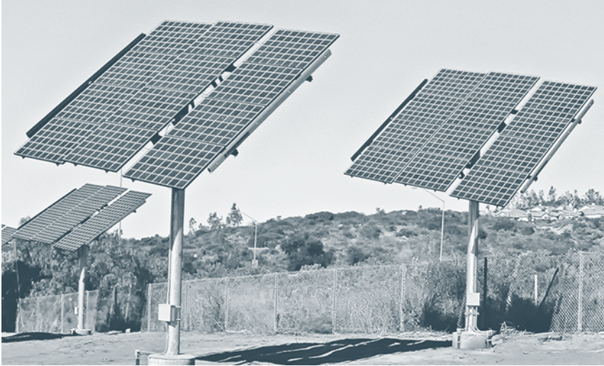
Figure 8.15. Passive Tracker. Passive trackers like this one do not require motors or photo sensors. How they work is explained in the text. Credit: Zomeworks.
