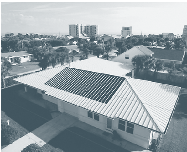
Figure 8.27. PV Laminate from Uni-Solar. PV laminate is applied directly to standing seam metal roof as shown here.
