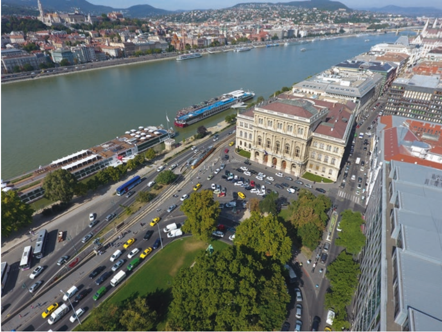
Fig. 5.13 Central building of the Hungarian Academy of Sciences
