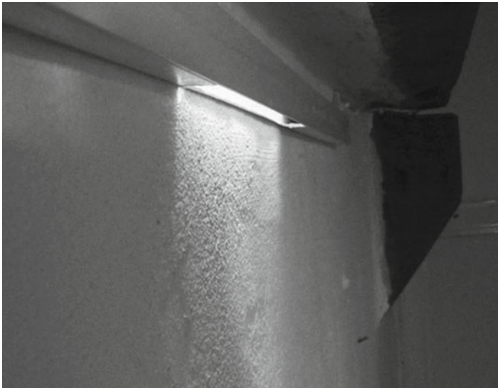
Figure 11-16. Light exit, cut into wire channel
