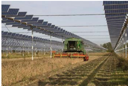
FIG. 6.2 View of an Agrovoltaico plant equipped with a dual-axis sun-tracking system [16].
