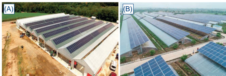
FIG. 6.22 (A) Solar PV panels mounted as a part of the roofs in commercial greenhouses implemented at Prides Corner Farms [106], and (B) The PV systems installed close to the greenhouses in Hongxingqiao Town, Changxing County, in east China's Zhejiang Province [107].
