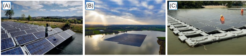
FIG. 6.3 (A) The FV system installed on an irrigation pond, Niente winery, California's Napa Valley region [25], (B) The FV system installed on a sandpit lake in Zwolle, the Netherlands [26], and (C) The FV system installed at Tengeh Reservoir in Tuas, Singapore [27].
