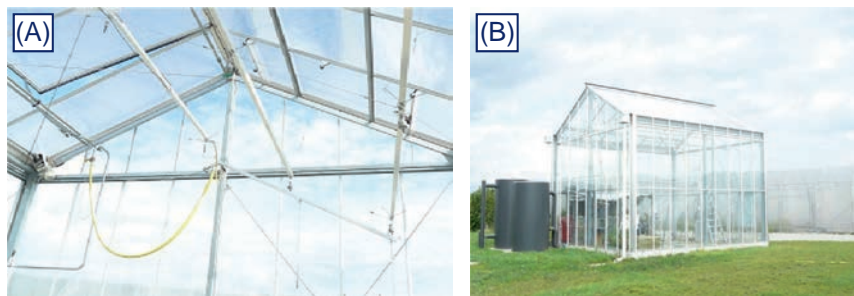
FIG. 6.26 (A) Linear Fresnel lenses and PVT modules integrated into a greenhouse hood, and (B) The solar greenhouse integrated with the CPVT module [125].
