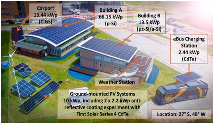
FIG. 11.17 The Fotovoltaica/UFSC solar lab, the 110kWp PV systems, and the eBus [66].
