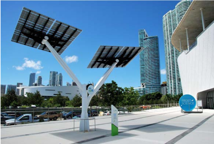
FIG. 11.23 Two lift solar tree project, Spotlight Solar Inc. [105].
