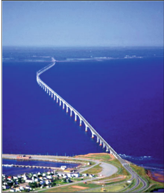
Fig. 14.8 Strength monitoring of a bridge with nanosensors. Image courtesy of IoN, UK
