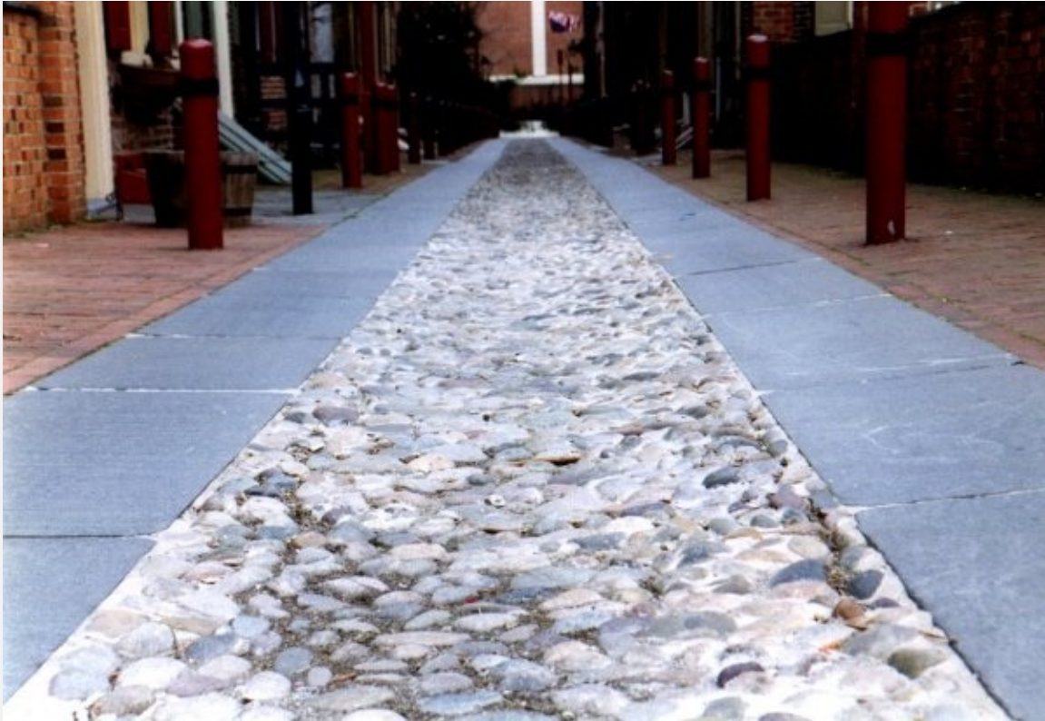
FIG. 3.15 Reconstruction of seventeenth-century cobblestone and pavement roadway, Elphreth's Alley, Philadelphia. Photograph by author.
