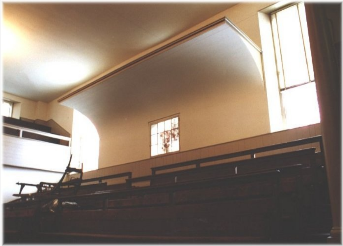
FIG. 3.16 One of the sounding boards above the facing benches in the Arch Street Meetinghouse, Philadelphia. Notice the width and height of the board, both of which serve to collect sounds from the whole room, including the galleries, in addition to projecting sounds. Photograph by author.
