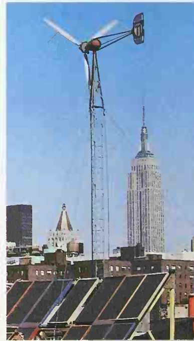
a propeller-type windmill on the roof of a city building, used to make electricity
