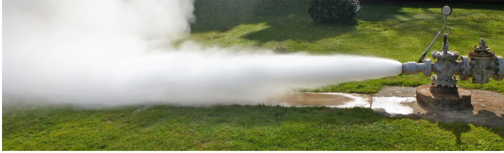
Figure 6.20 Horizontal atmospheric discharge of a direct use well without a lip pressure pipe (Rotorua, New Zealand). Picture by authors.
