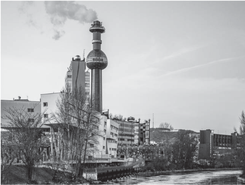
Figure 5.15 Spittelau Waste Incineration CHP plant in Vienna, on the Danube River. Source: © Soysal.
