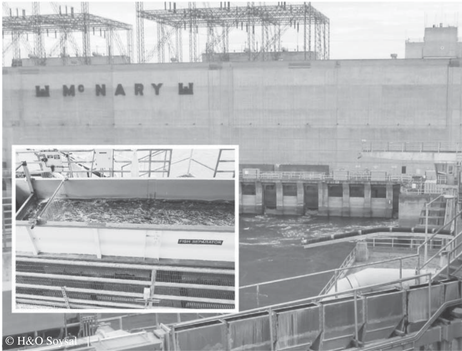
Figure 5.5 Fish separation facility at McNary Dam, Oregon. Source: H. & O. Soysal.
