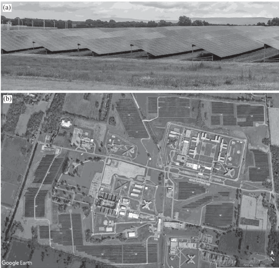
Figure 10.10 Solar farm near Hagerstown, Maryland, US. (a) Ground-mounted PV arrays. (b) Satellite view of the 1.1-MW capacity CES VMT solar farm operated by Consolidated Edison Solutions Inc. Source: Image captured from Google Earth on 6/29/2019.
