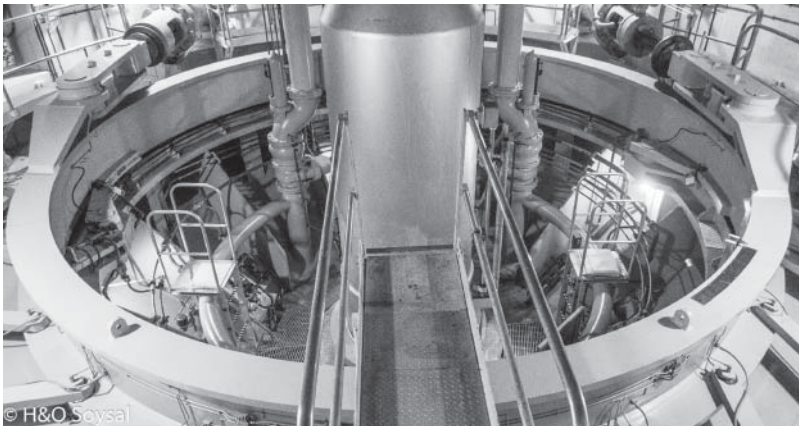
Figure 8.6 Wicket gates control mechanism during maintenance at Bonneville Dam, Oregon.
