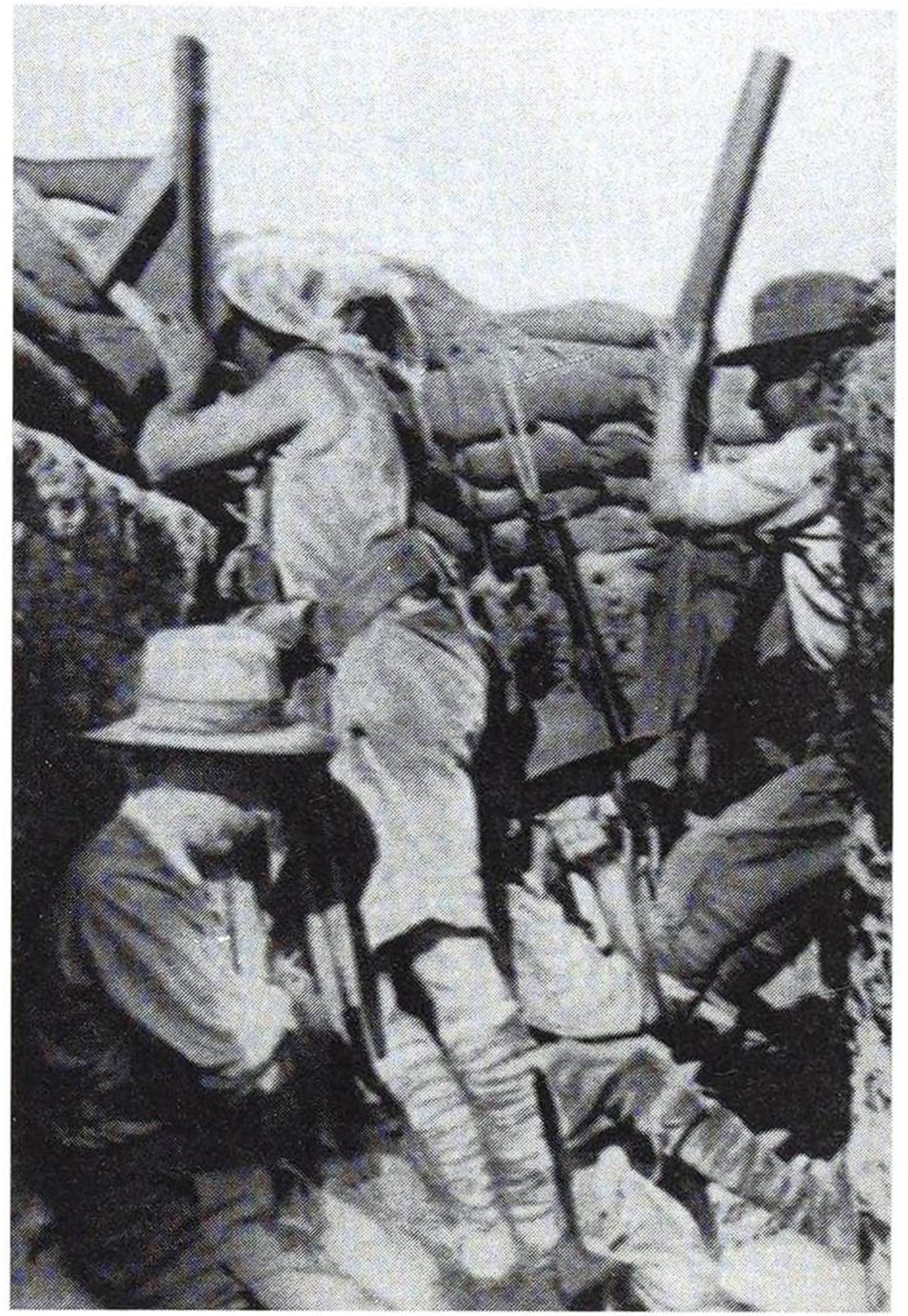
An even simpler Royal Engineers sniperscope used in the Dardanelles. The periscope forms the back of the device. The trigger is pulled by a wire. The man behind the shooter is observing with a locally made periscope. (The Times History of the War)
