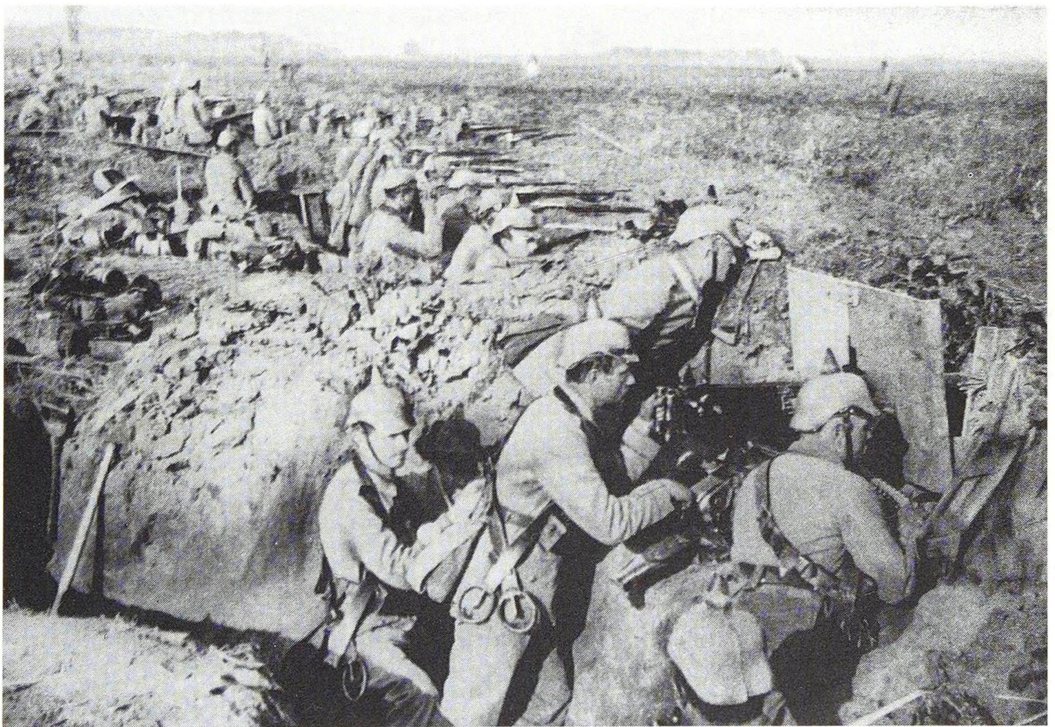
German trench, late 1914. The machine-gun crew are using a trench shield. Note the outward curvature of the sides to prevent bullet splash causing injuries. (The Illustrated War News)
