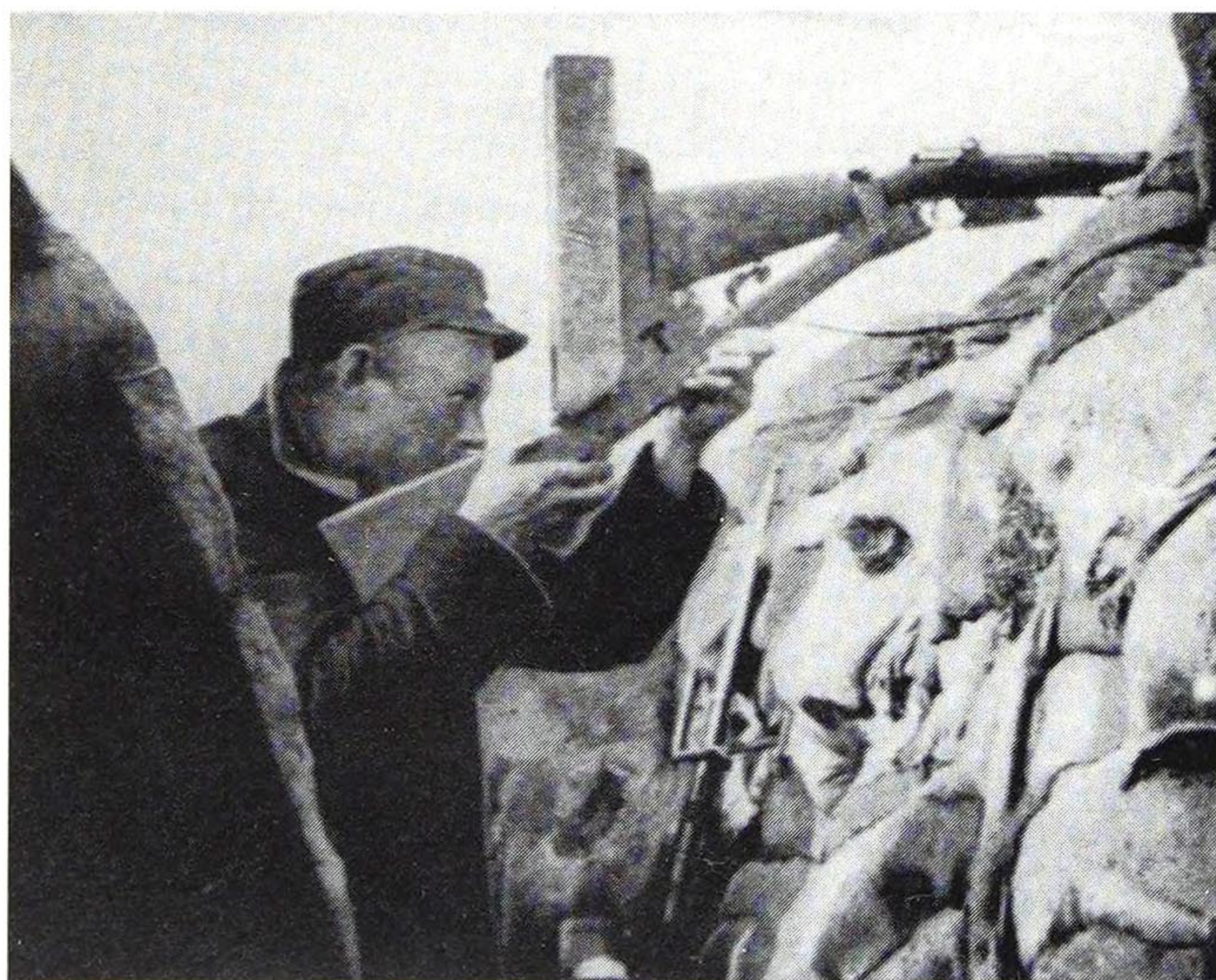
A Belgian sniperscope with auxiliary trigger, 1915. Although this appears to be a simple, robust device, it does not allow the shooter much cover. (The Times History of the War)
