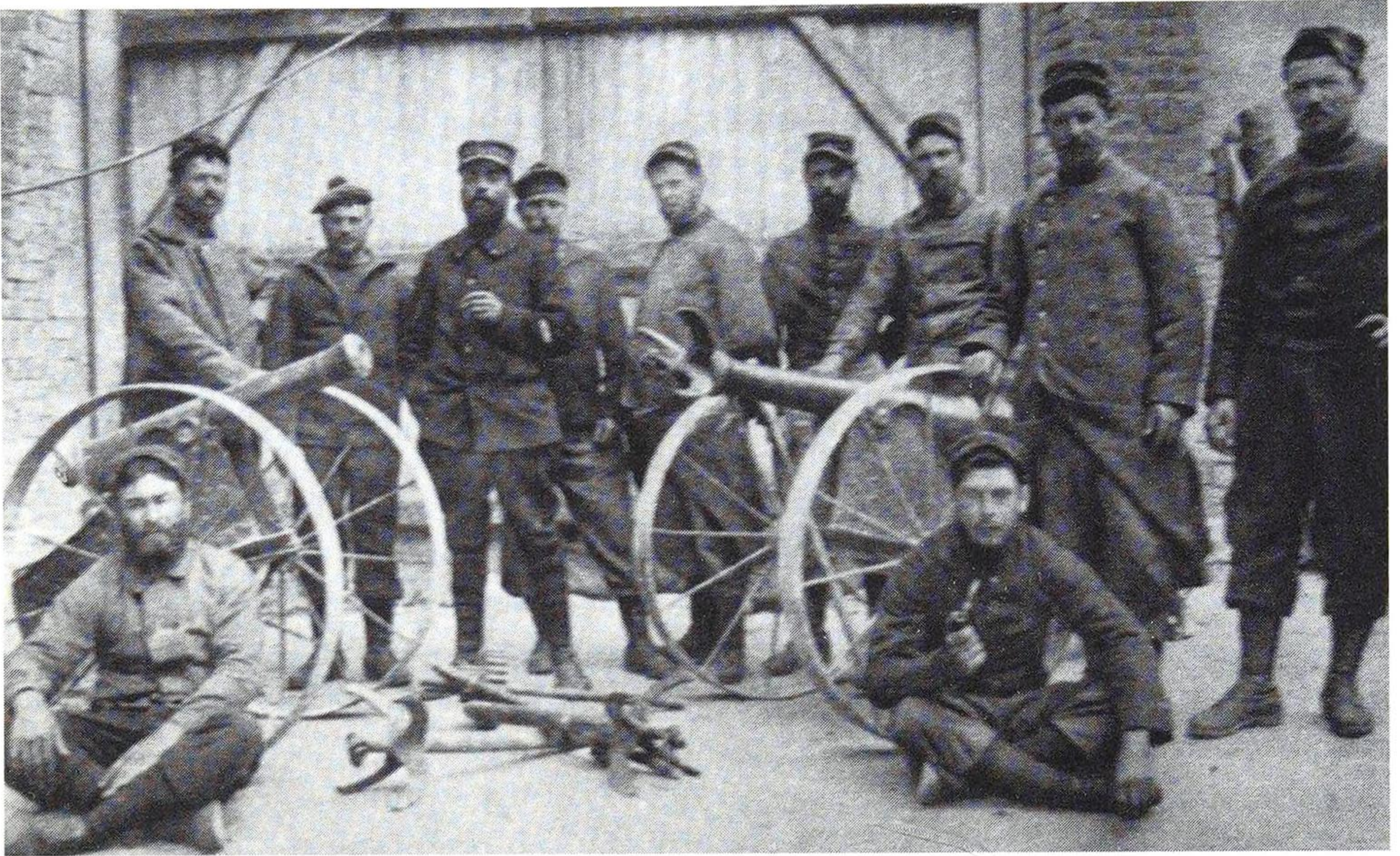
A group of French artillerymen pose with ancient cannon used for firing the grapnels that are displayed in front of them, summer 1915. The grapnels, attached to ropes or chains, are fired into wire entanglements then reeled back through the entanglement to clear a path – at least, in theory. (The Illustrated War News)
