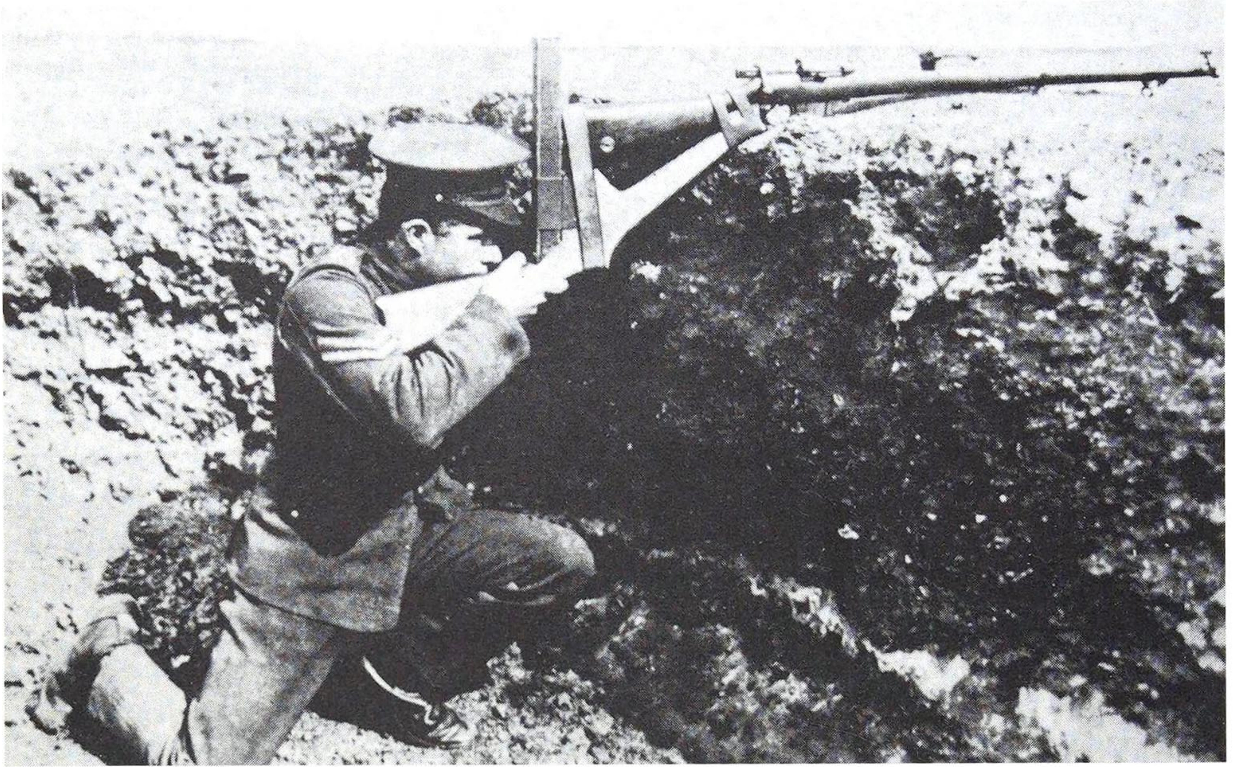
An early sniperscope constructed by Mr Walker of the Birmingham Small Arms Co. for his son who was serving in the 6th Warwicks. Although from the way the shooter is holding the auxiliary stock, it appears to be fitted with an auxiliary trigger, it is not. The rifle's trigger has to be operated with the left hand. Again, the device offers only minimal cover but the recoil was reported to be less than expected. However, the muzzle jumped by about 1.5 in. (The Illustrated War News)
