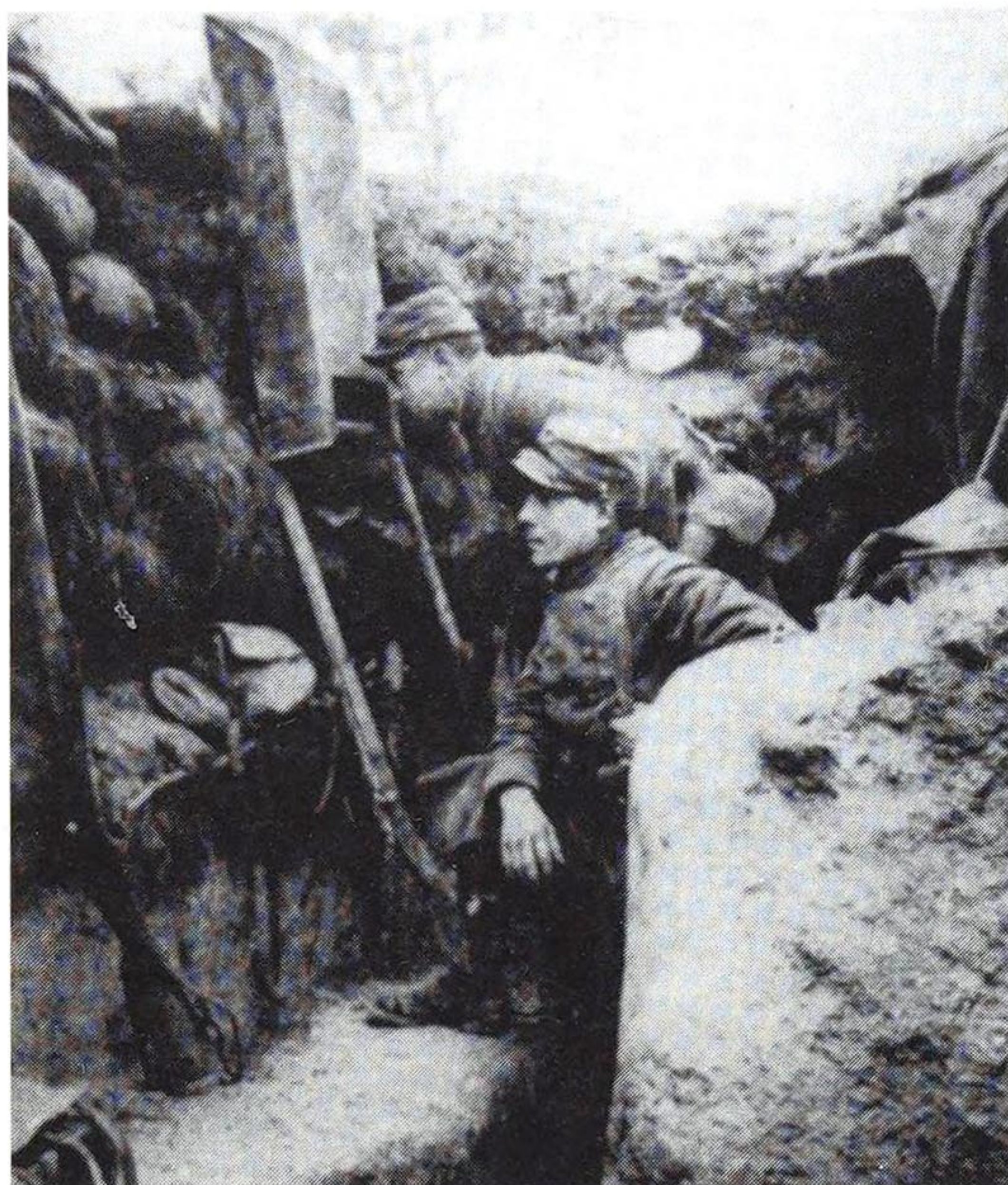
A French box periscope with wide mirrors, 1915. (The Illustrated War News)
