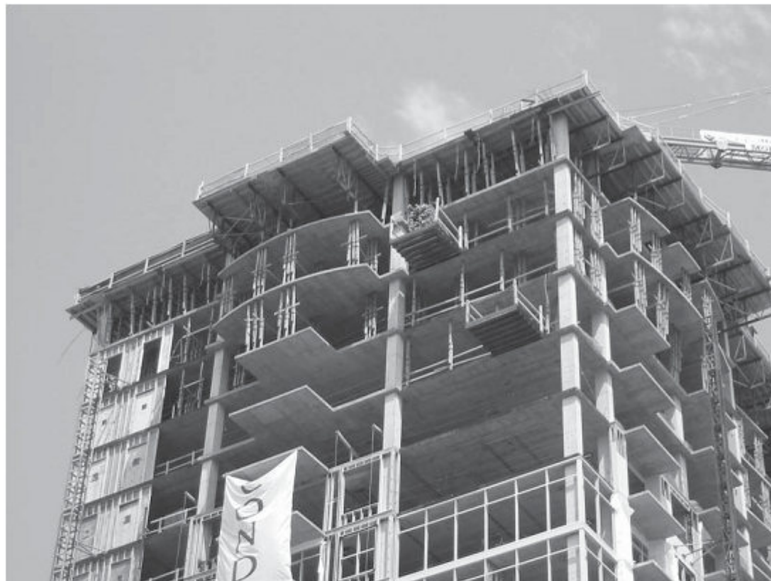
Flat Plate Construction—Pharr Road Condominiums, Atlanta, Georgia.
