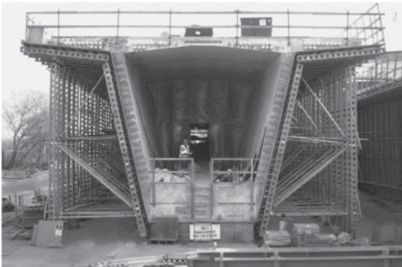
Pre-cast segments for the I-35W St Anthony Falls Bridge, Minneapolis, Minnesota.
