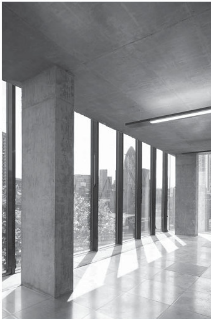
Flat plate without edge beams. (Buckley Gray Yeoman, Fashion Street, London, 2010)
