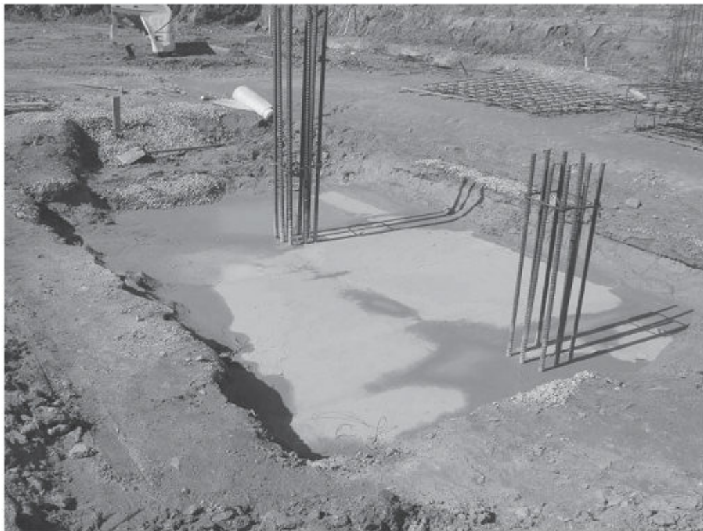
Combined footing (two column) after footing concrete is placed showing column reinforcing bars ready for splicing.
