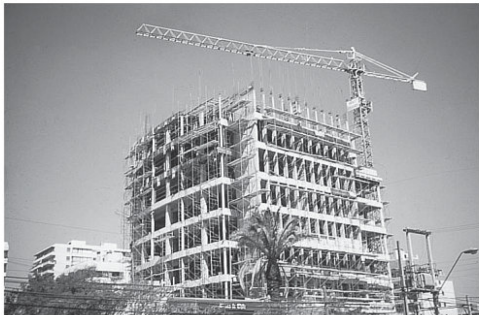
The 16-story Apoquindo Tower, Santiago, Chile.
