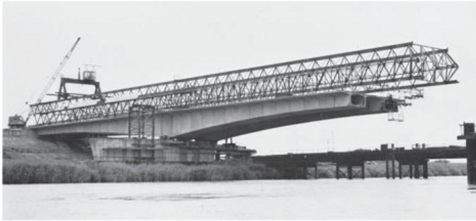
Prestressed concrete segmental bridge over the River Trent near Scunthorpe, Lincolnshire, England.
