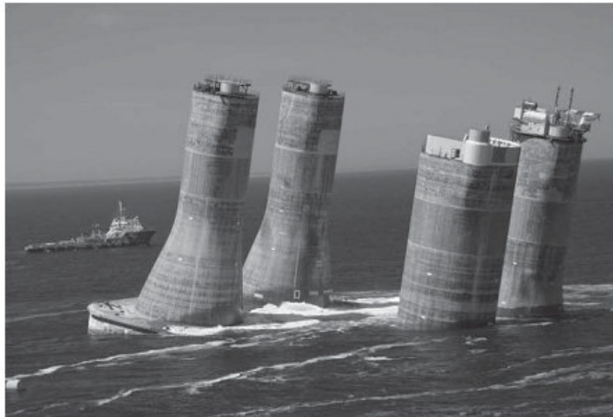
Installation of the concrete gravity base substructure (CGBS) for the LUNA oil-and-gas platform in the Sea of Okhotsk, Sakhalin region, Russia.
