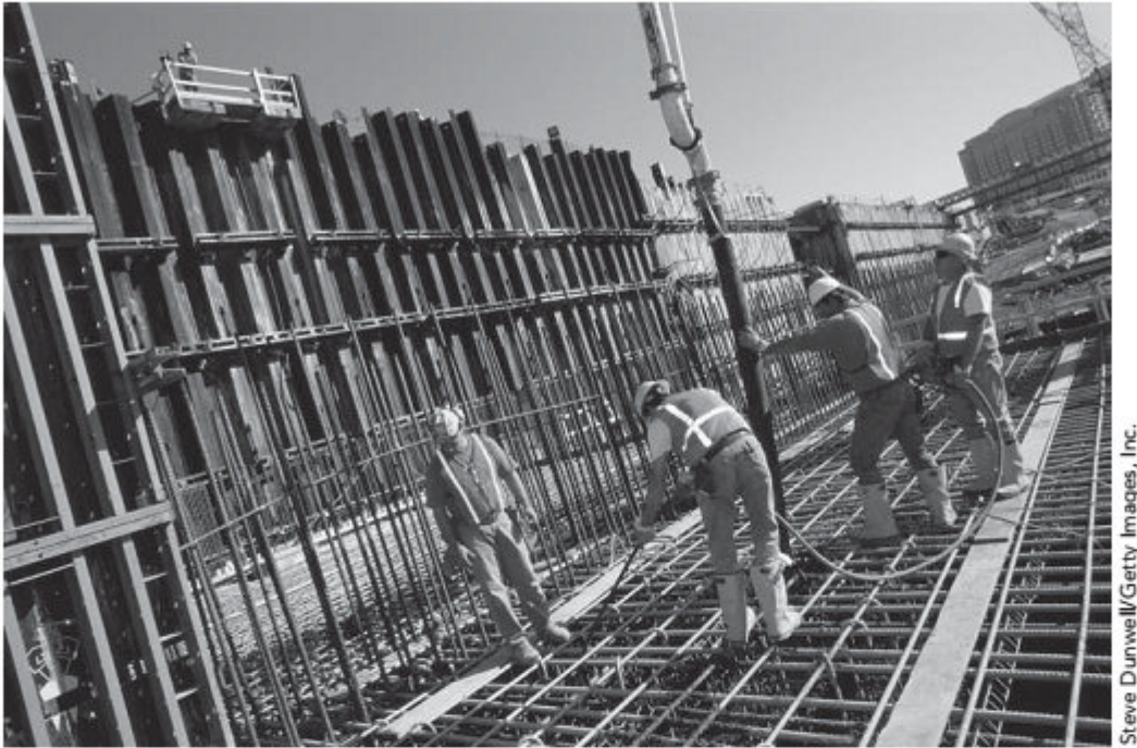
Pouring concrete, Big Dig, Boston, Massachusetts.
