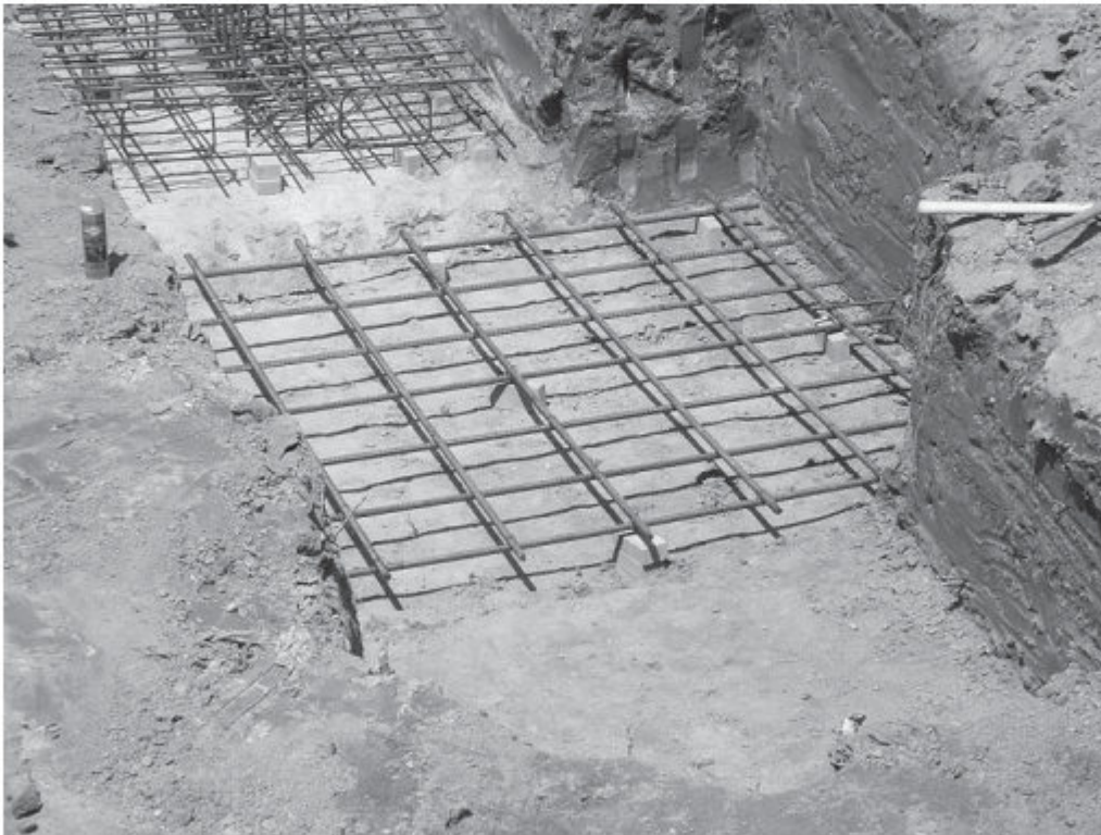
Single-column footing prior to placement of column reinforcing bars.
