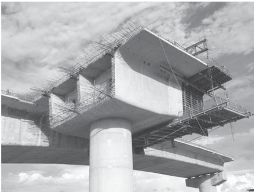
Segmental prestressed concrete bridge construction.
