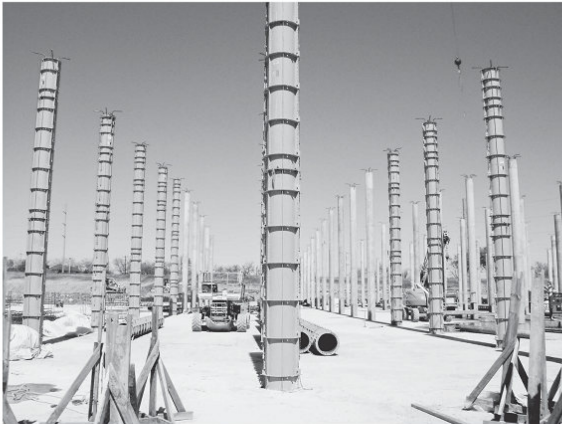
Columns of variable heights between 25' and 35' will provide support for tank lids for the Eastside Treatment Plant in Sunnyvale, Texas.
