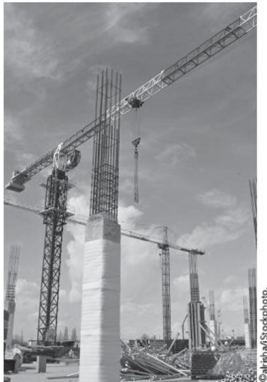
Reinforced concrete columns.
