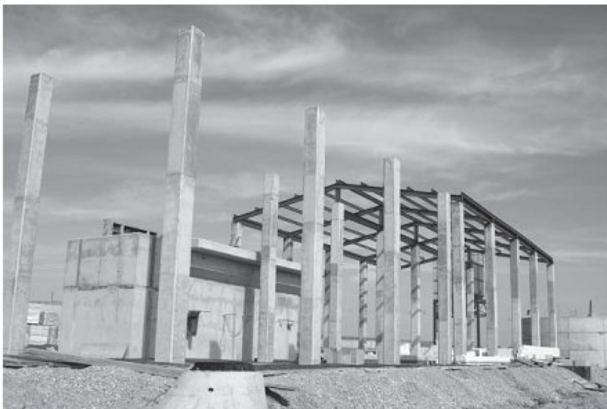
Reinforced concrete columns and shearwalls supporting structural steel roof.
