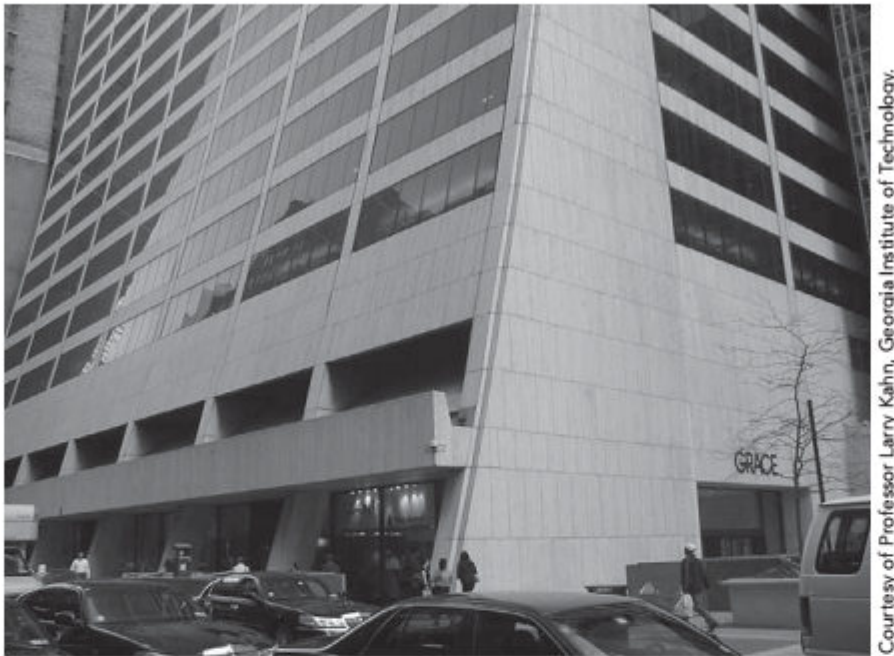
Buttress shear wall, Grace Building, New York, NY.
