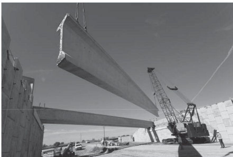
Prestressed bridge girders during erection.
