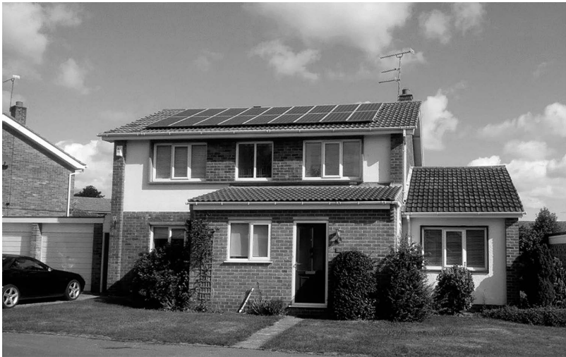
FIGURE 7.2 The MyGridGB home with 3.6 kWp of rooftop solar panels and battery energy storage. Modern technology means that the existing solar array could be 50% more powerful, and batteries could have twice the capacity for less capital than was originally spent on just the solar array.
