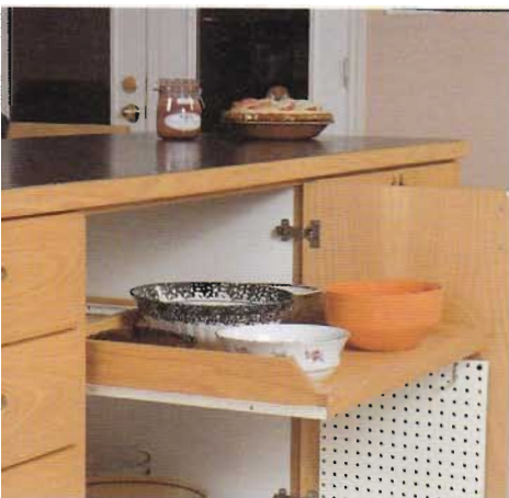
Pull-out shelves are a combination of shelves and drawers. Instead of searching through a stack of pots and pans in your lower cabinets, just slide out the shelf and pick what you need. Build your own using drawer slides.
