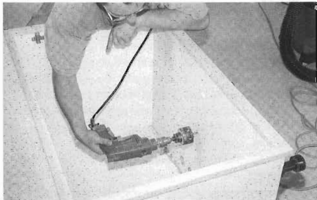
Fig. 6-14 Plumbing and the possibility of water leaks inside this cabinet should be taken into account when designing the sink base.
