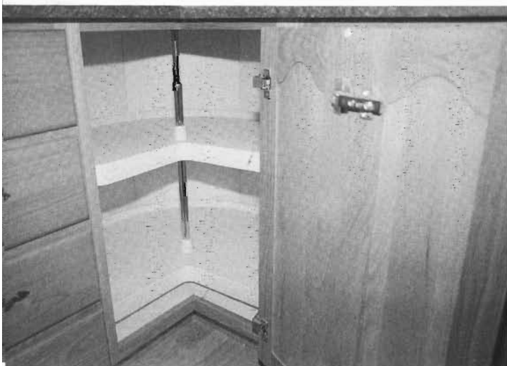
Fig. 1-13 36" corner base cabinet with 32" pie-cut lazy susan installed
