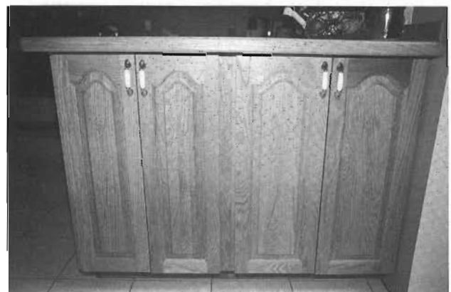
Fig. 1-11 Solid-core hardwood cabinet doors are often the most expensive type of door.
