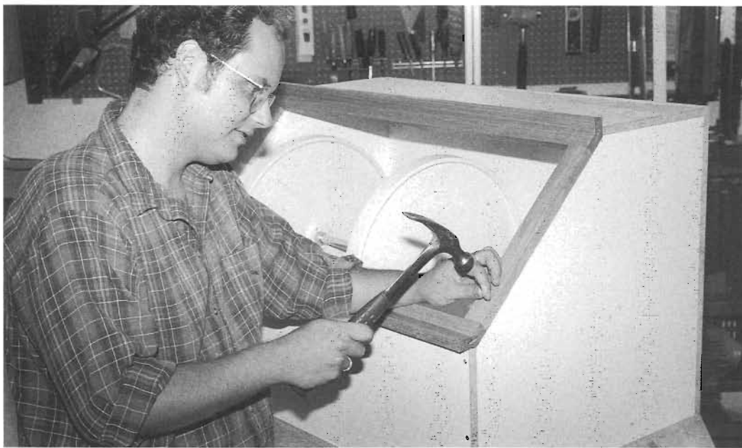
Fig. 5-14 Installing the face frame on the upper corner cabinet
