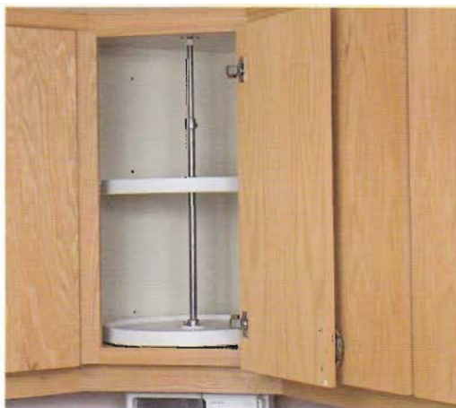
Utilize wasted corner space by installing a lazy susan. In upper cabinets, use a regular corner cabinet with 170° full-overlay hinges.
