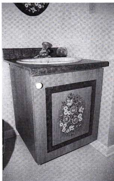
Fig. 1-28 A modified-height base cabinet was built for this basement bathroom. The toe kick board was not installed because of the danger of water on the floor. Because this cabinet has plastic adjustable legs, the possibility of water damage has been eliminated.
