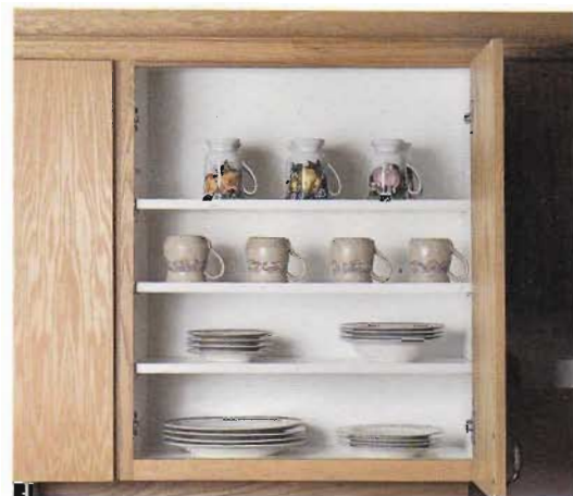
Perhaps the simplest innovation for customizing your cabinets and maximizing storage space is adjustable shelving. You can change shelf heights to accommodate what you are storing, and when you want to rearrange the kitchen, it is as simple as moving a few shelf pins.
