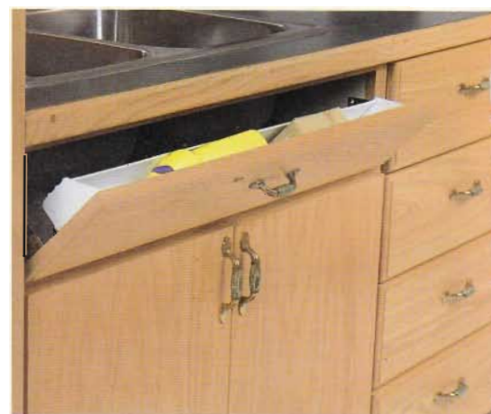
Many times kitchen cabinet-makers put a false drawer front in front of the sink so that it matches the rest of the drawers and cabinets. Why not use the four or five inches of dead space under the cabinet for a flip-out to store dish soap, sponges and other small items?
