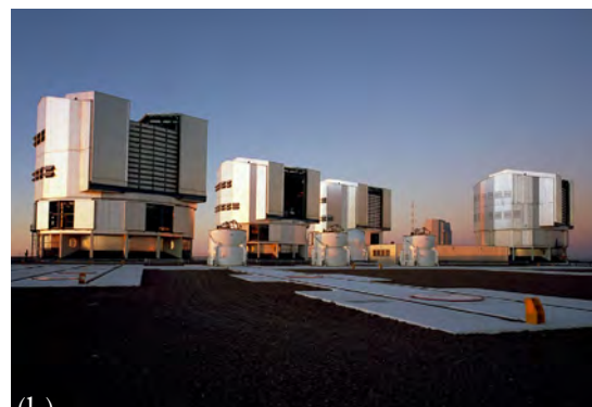
Figure 7.7. Light signals from multiple telescopes can be combined through interferometry to increase the resolution of the image, as is done at the Very Large Array (left) and the Very Large Telescope Interferometer (right). VLT image courtesy of NRAO/AUI. VLT image courtesy of ESO/H.H.Heyer.
