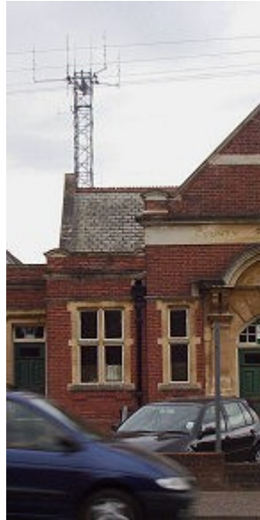
TETRA on North Walsham police station, Norfolk.
