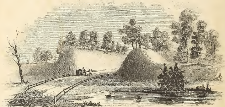
FIG. 20.—VIEW OF GRADED WAY NEAR PIKETON, OHIO.
