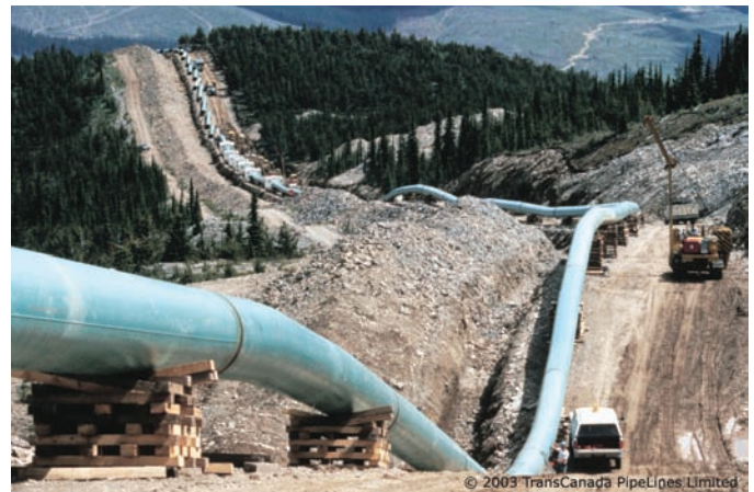
Fig. 2-21 Cross-country pipeline being made. Note the rugged terrain. The pipe cannot be rotated so much to be welded in position. Both 5G and 6G would be common. The 6G welds are often referred to as “Arkansas Bell Hole.” © TransCanada Pipelines Ltd.
