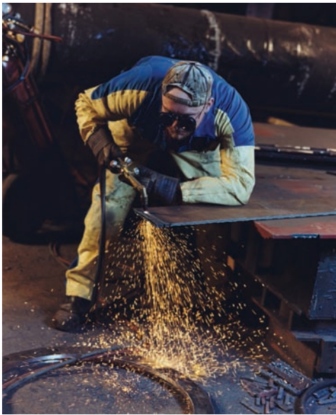
Fig. 6-2 Cutting bar stock which is part of the structural steel on a building construction job. © Johner Images/Getty Images
