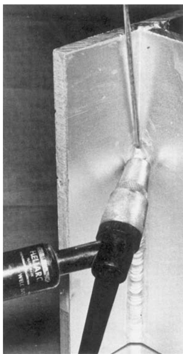
Fig. 19-31 Positions of the torch and filler rod when making a vertical fillet weld in aluminum plate. © Kaiser Aluminum
