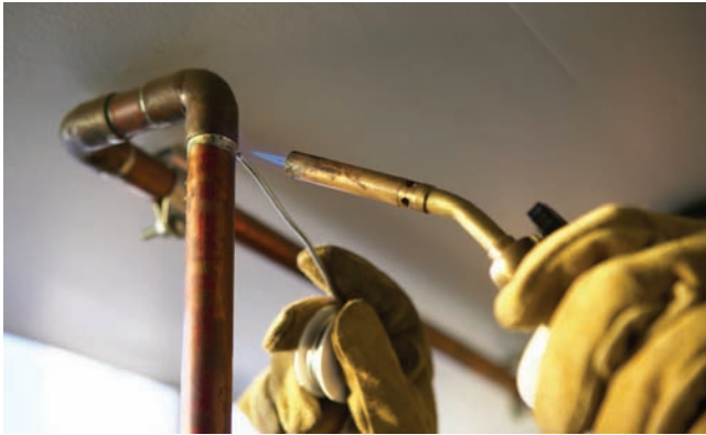
Fig. 10-1 Soldering a copper tube with a butane torch. © Prographics
