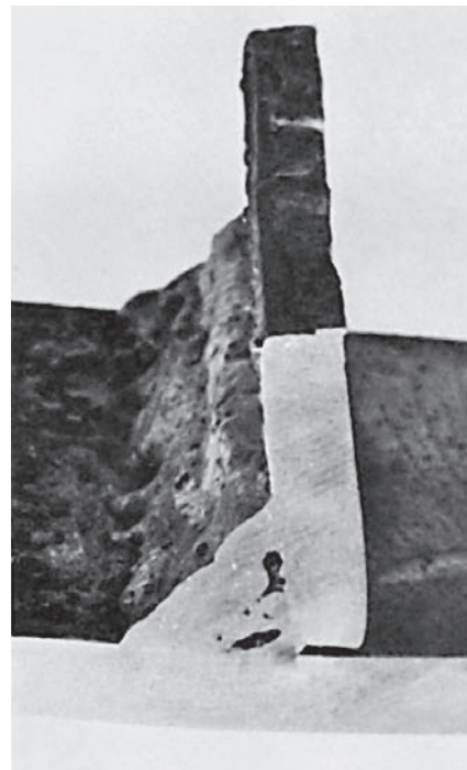
Fig. 28-106 Cross section of a fillet weld, exposing internal defects caused by slag inclusions in the weld metal deposit. These voids reduce the mechanical properties of the weld metal.
