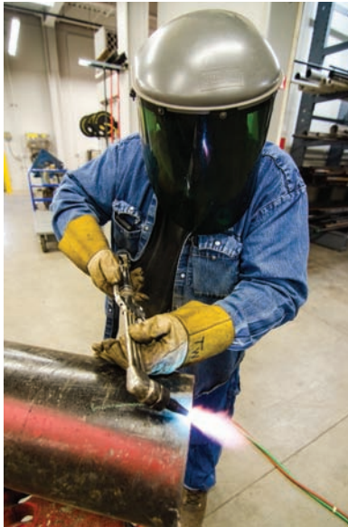
Fig. 16-94 Welding apprentice using an oxyacetylene hand cutting torch to flame cut and bevel pipe. A great deal of field fabrication is cut with this method. Location: UA Local 400 © McGraw-Hill Education/Mark A. Dierker, photographer
