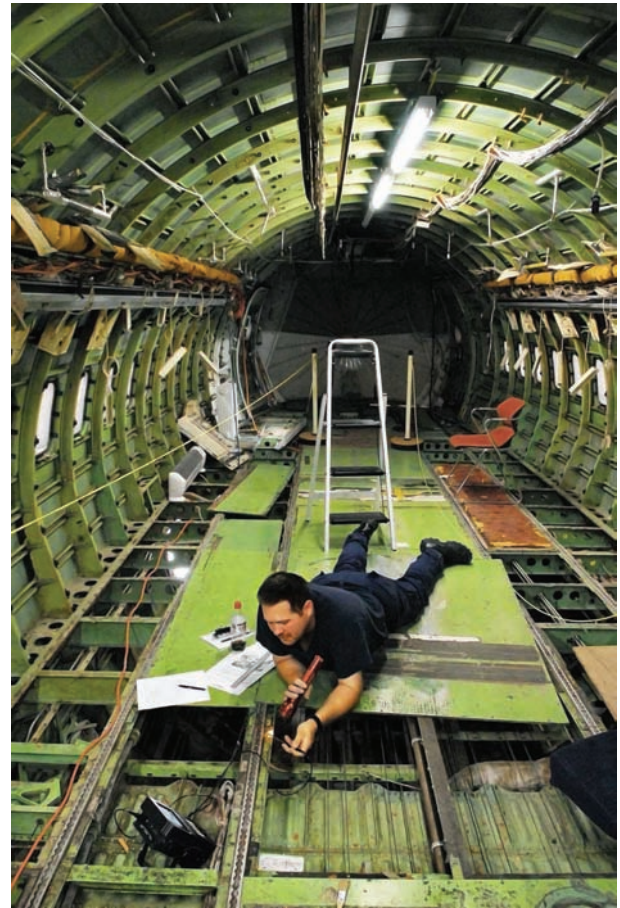
Fig. 28-49 Eddy current testing for industrial applications requiring surface and subsurface crack detection and metal sorting. This method and equipment can deliver productivity, quality, and safety in a very portable unit. Randy Montoya/US Coast Guard
