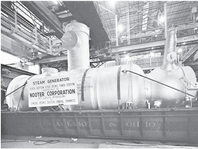
Fig. 2-33 This steam generator plant has a capacity of 127,000 pounds and contains more than 9 miles of tubing. The plant produces steam from controlled nuclear fission. © Nooter Corp.
