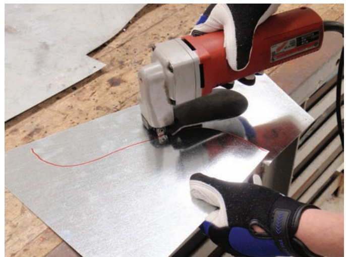
Fig. 26-62 Using a portable electric shear on a 16 gauge galvanized sheet metal. It can be used for straight line, curved lines or circle cutting. The cutting speed is 10 feet per minute. © Renee Bohnart
