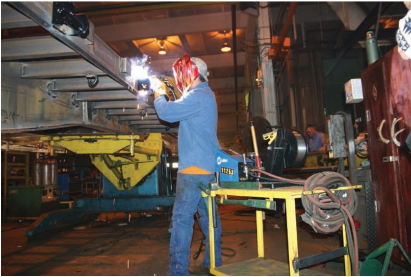
Fig. 21-1 GMAW being performed on a carbon steel trailer frame. Note the positioner, which is able to optimize the welding into flat and horizontal positions. © Miller Electric Mfg. Co.
