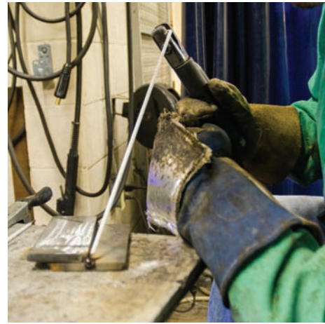
Fig. 13-2 Student welder is making a fillet weld on a lap joint. Seated at a workbench in order to be as relaxed and comfortable as possible. Note that they are wearing required protective gear. Location: Northeast Wisconsin Technical College © McGraw-Hill Education/Mark A. Dierker, photographer
