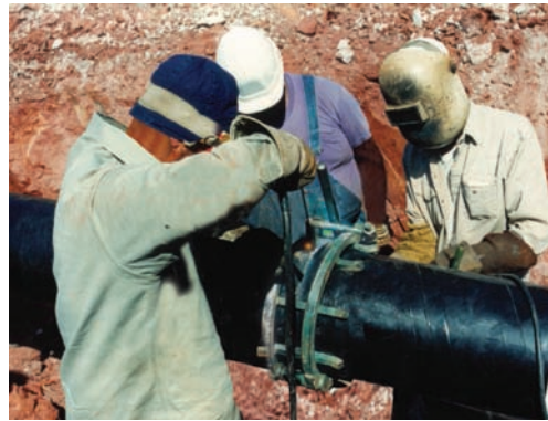
Fig. 16-24 Clamps are available in several types and models from 2- to 60-inch diameters. This type of cage clamp is fast and efficient when only alignment is required. © Mathey Dearman
