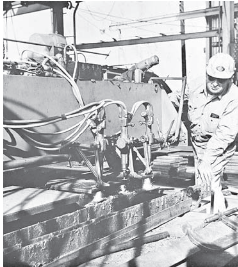
Fig. 2-41 All of the fabrications shown in this chapter used gas and arc cutting as a fabricating tool. Shown here is a multiple-torch application, burning natural gas and oxygen, which is cutting out parts that will later become part of a weldment. © Praxair, Inc.
