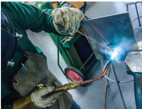
Fig. 8-19 Welding in the vertical position. Location: Northeast Wisconsin Technical College © McGraw-Hill Education/Mark A. Dierker, photographer
