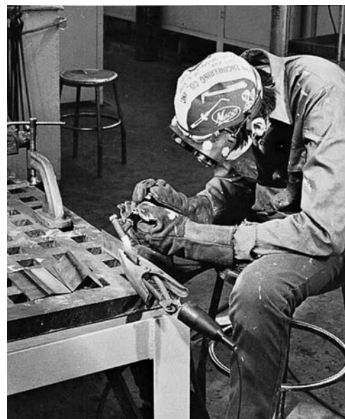
Fig. 18-65 Making an edge joint with the plasma needle arc.
