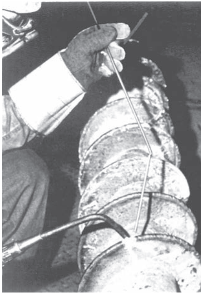
Fig. 9-14 Welder uses oxyacetylene torch and Haynes-Stellite no. 6, a hard-surfacing rod, to hard surface edges of a screw conveyor for handling crushed limestone. © Praxair, Inc.
