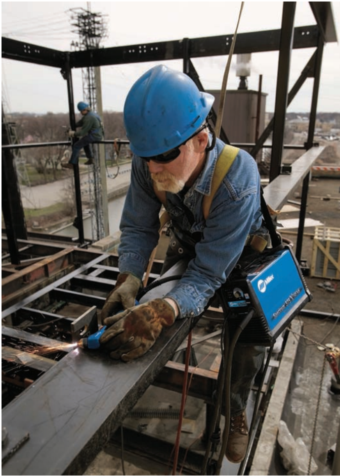
Fig. 17-11 Cutting a carbon steel plate manually with the plasma arc process and very portable power source. The process has the same flexibility as oxyacetylene without the large cumbersome cylinders. Note the protective clothing and fall restraint. © Miller Electric Mfg. Co.
