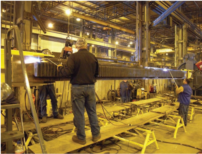
Fig. 23-3 Prior to welding, this is a more than 25-foot-long rack gear for a large capacity crawler crane. There will be approximately 100 feet of \frac{5}{8} -inch weld size J-groove weld on this project when completed. The plate and weld areas will be preheated to 500°F, and it will take approximately 20 hours to complete the fabrication. With careful execution of the preheat, welding procedure with staggering and skip welding techniques twist and flatness was maintained over its length to less than \frac{1}{2} the electrode diameter. Head and tail stocks were used to position the welds in the flat position. © The Manitowoc Company, Inc.
