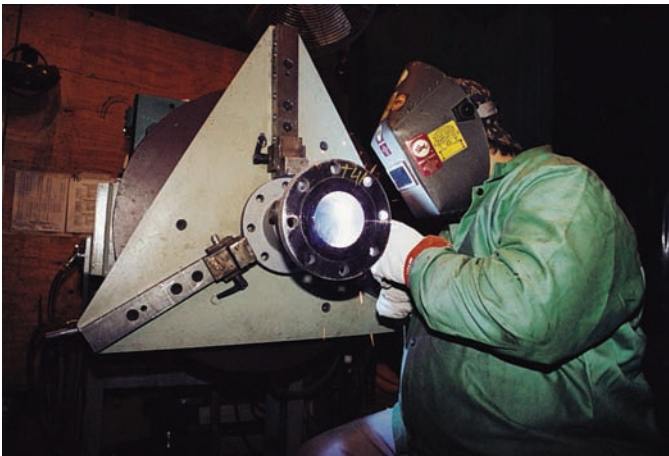
Fig. 24-3 Welding carbon steel pipe in the shop with the GMAW short circuit mode of metal transfer on the root pass. Note the arc visible on the inside of the pipe. This ensures that complete penetration is taking place. A pipe gripper is attached to a turning fixture that is rotating the pipe. © Miller Electric Mfg. Co.
