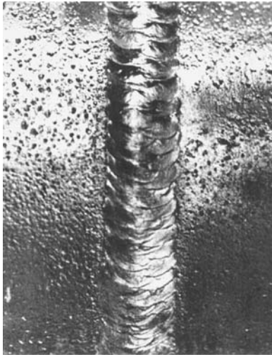
Fig. 24-13 Sample of a weaved finish pass on a butt joint in pipe welded in the roll position. © Plumbers and Pipefitters Union, Alton, IL
