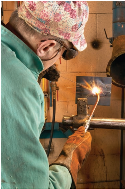
Fig. 8-21 Welding in the horizontal position on steel plate. Note torch and filler rod angles. © Prographics
