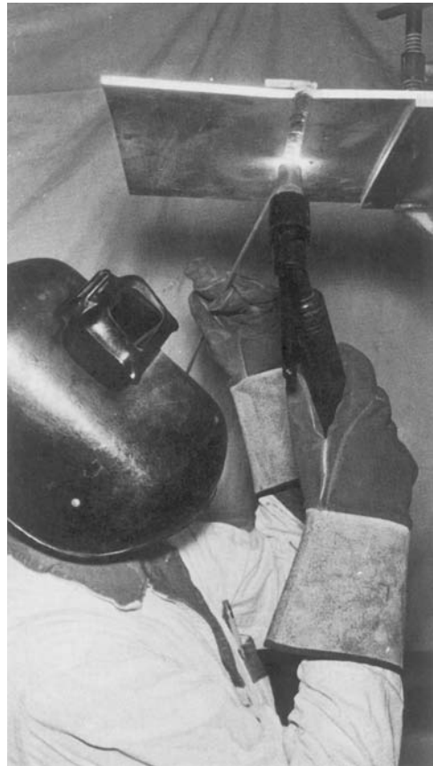
Fig. 19-38 Positions of the torch and filler rod when welding a butt joint in the overhead position in aluminum plate. © Kaiser Aluminum
