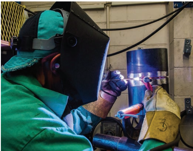
Fig. 20-33 A properly cleaned pipe inside and out being tacked together. The pipe axis in the vertical orientation. The weld will be made in the horizontal (2) position. Filler metal is being used on this V groove weld on a butt joint. Location: Northeast Wisconsin Technical College © McGraw-Hill Education/Mark A. Dierker, photographer
