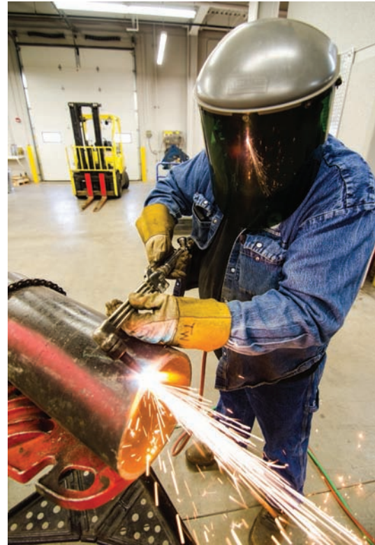
Fig. 7-35 Making a manual bevel cut on a pipe. As might be required in the field. It would be impossible to find a shape that could not readily be cut with the handheld cutting torch. Location: UA Local 400 © McGraw-Hill Education/Mark A. Dierker, photographer
