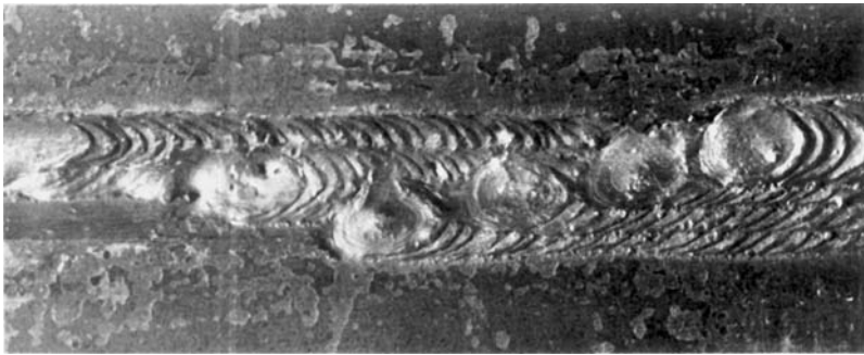
Fig. 15-49 V-groove butt test joint with a backing bar and a 1/4-inch root opening welded in the horizontal position (2G). Note the sequence of weld beads and the appearance.
