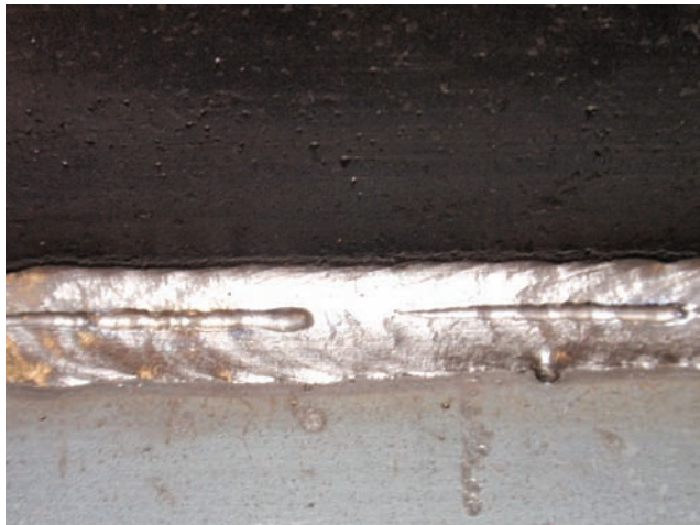
Fig. 21-66 A fillet weld made with the flux core process. Note the elongated surface porosity (worm tracks) due to contaminated wire and or too little electrode extension. © Edward R. Bohnart
