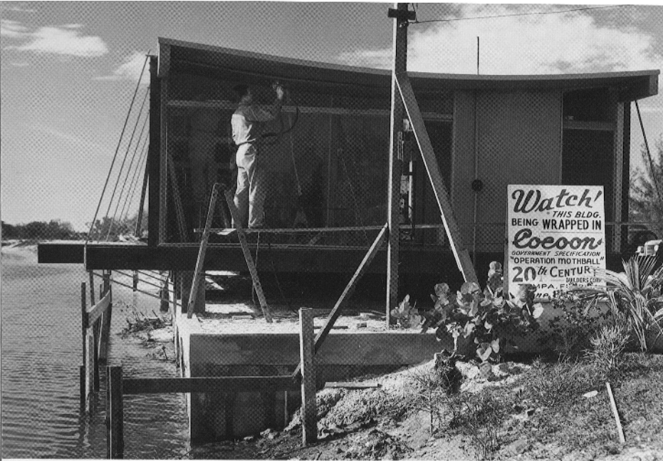
HEALY GUEST HOUSE (COCOON HOUSE), UNDER CONSTRUCTION
