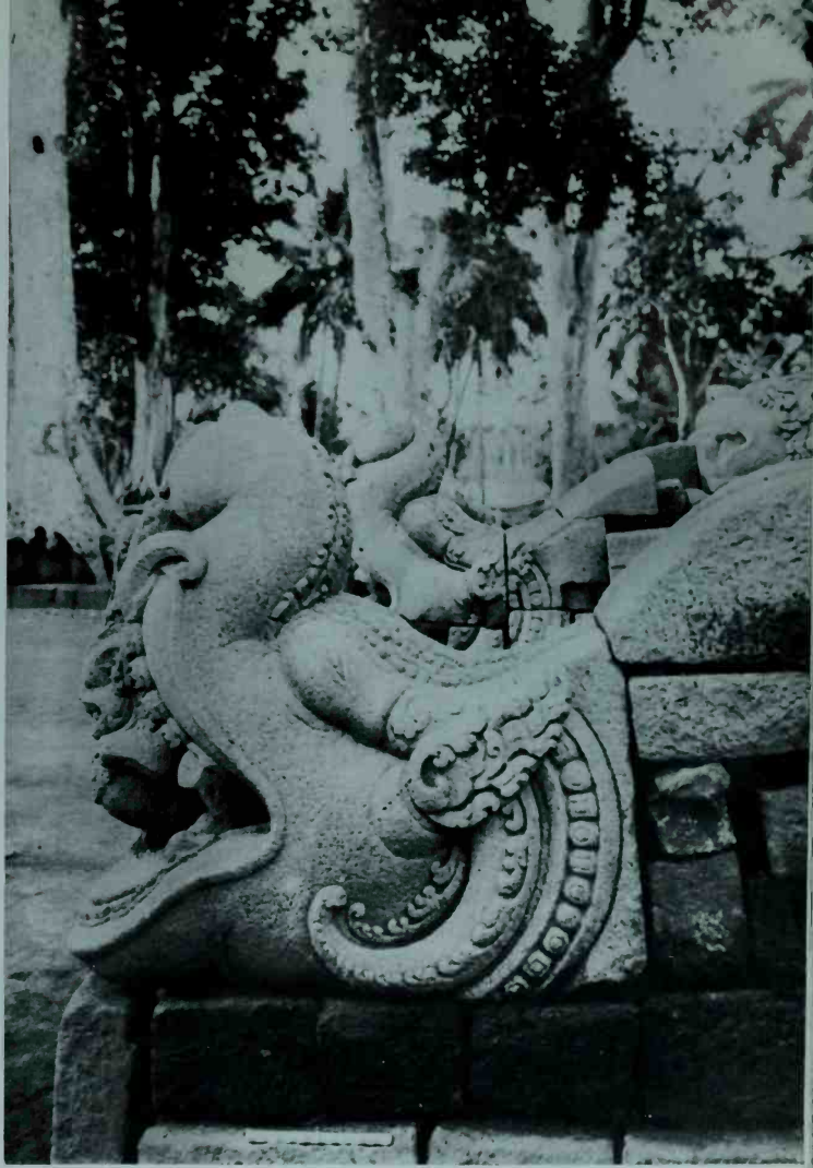
189 Borobudur, a makara terminal. These monster- heads terminate the stair balustrades
