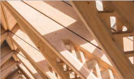
The lattice beam structure is made using Nordic spruce
