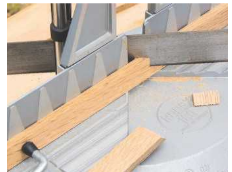
STEP 12. Cut the top and bottom panels to size. Prepare 10mm-thick lipping and mitre the ends of each strip
