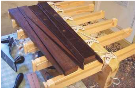
STEP 42. The wedge and lace jig is made from building timber and hardwood
