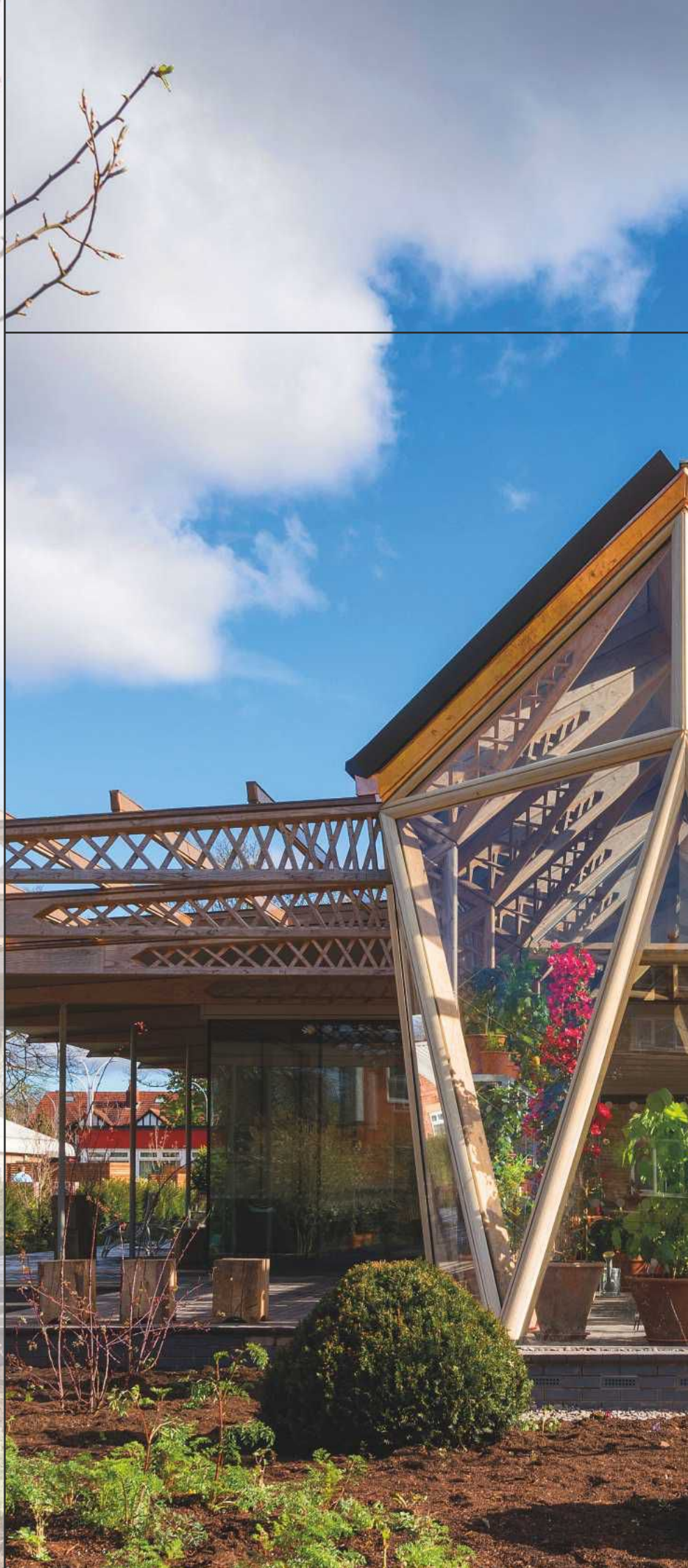
The roof is naturally illuminated by triangular roof lights and is supported by lightweight timber lattice beams
