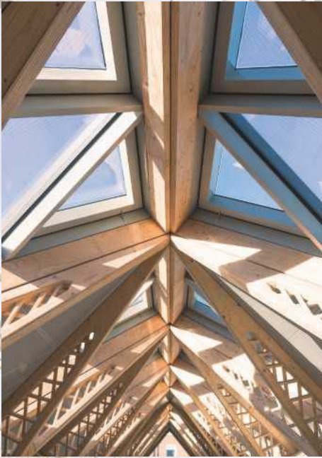
The roof is naturally illuminated by triangular roof lights and is supported by lightweight timber lattice beams
