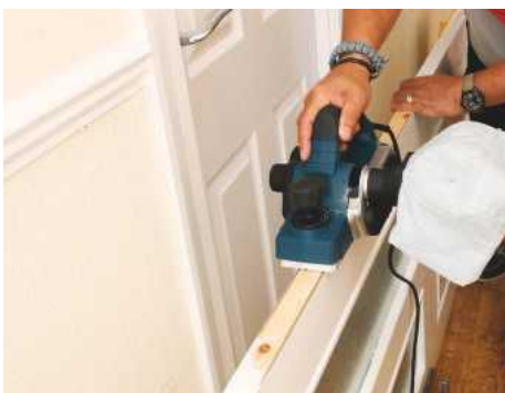
Easing and fitting doors are bread and butter work for this planer
