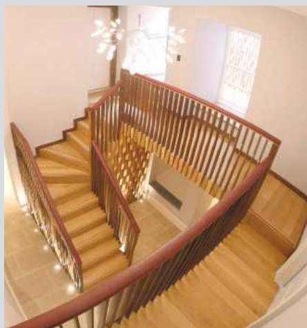
The spindles of the staircase are cut with arcs of varying sizes to create an organic flow
