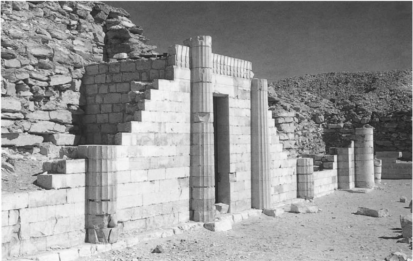
Fig. 10. Facade, South House
