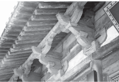
FIGURE 3.9. Bracketing under front eave of the Soul-Sleeping Hall at the Shrine for the God of the Ji River in Jiyuan, Henan: note identity between the column sets and the intermediate sets, both of five puzuo with two layers of protruding arms, having no lateral arms on the lower layer (author photograph)
