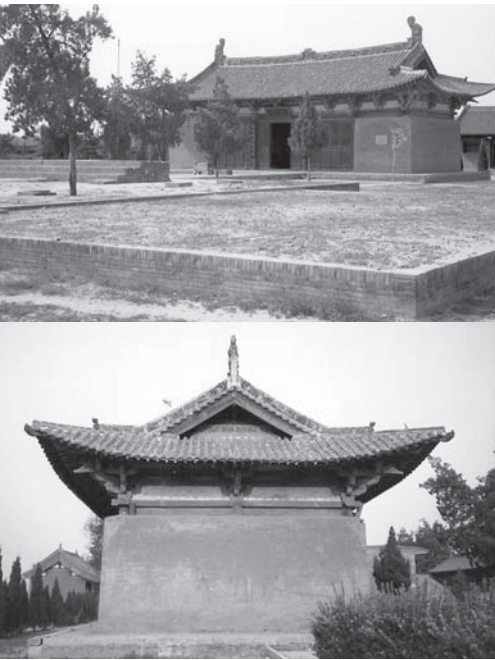
FIGURE 3.8. Soul-Sleeping Hall at the Shrine for the God of the Ji River in Jiyuan, Henan, with Song beam structure and bracketing (built 973): (top) front view; (above) side view (author photograph)
