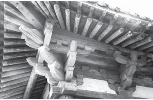
FIGURE 3.10. Corner bracket sets in the Soul-Sleeping Hall at the Shrine for the God of the Ji River in Jiyuan, Henan, featuring intersected arms from two directions ( liegong ), “mandarin-duck head-crossing” arms ( yuanyang jiaoshou gong ), pupaifang supporting all sets and stretching their heads from two directions, and the “head-raising” timber ( shengtoumu ) facilitating the eaves’ turning upward (author photograph)
