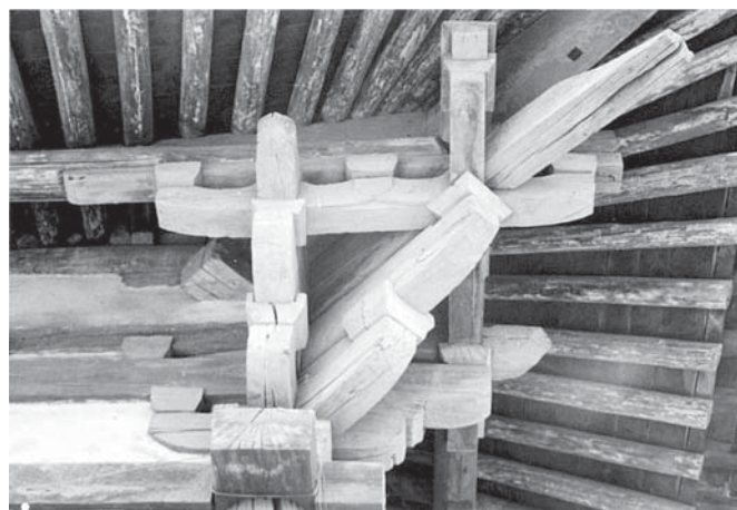
FIGURE I.3. Bracketing of the Soul-Sleeping Hall (973) at the Shrine for the God of the Ji River in Jiyuan, Henan (featuring a corner bracket set, front and upward view; author photograph)
