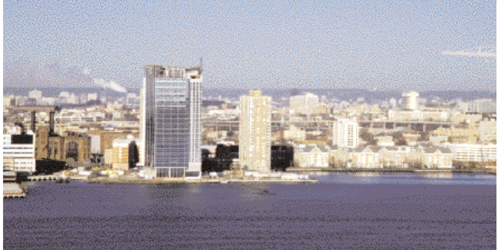
5. HARBORSIDE PLAZA X UNDER CONSTRUCTION, JERSEY CITY, NEW JERSEY, 2002, HLW INTERNATIONAL
