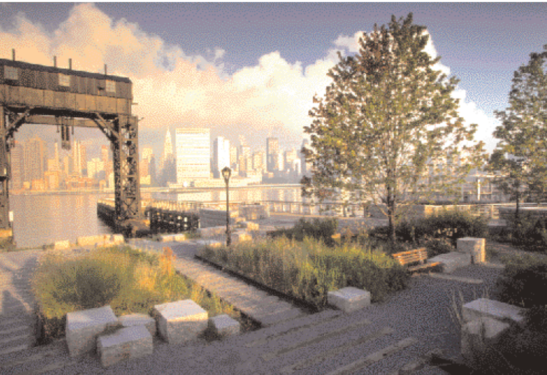
23. GANTRY PLAZA STATE PARK, QUEENS WEST, LONG ISLAND CITY, QUEENS, 1998, THOMAS BALSLEY ASSOCIATES, SOWINSKI SULLIVAN ARCHITECTS, WEINTRAUB & DI DOMENICO
