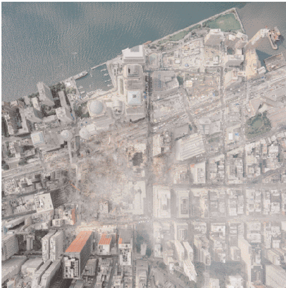
2. AERIAL VIEW FROM DIRECTLY ABOVE WORLD TRADE CENTER SITE, SEPTEMBER 2001
