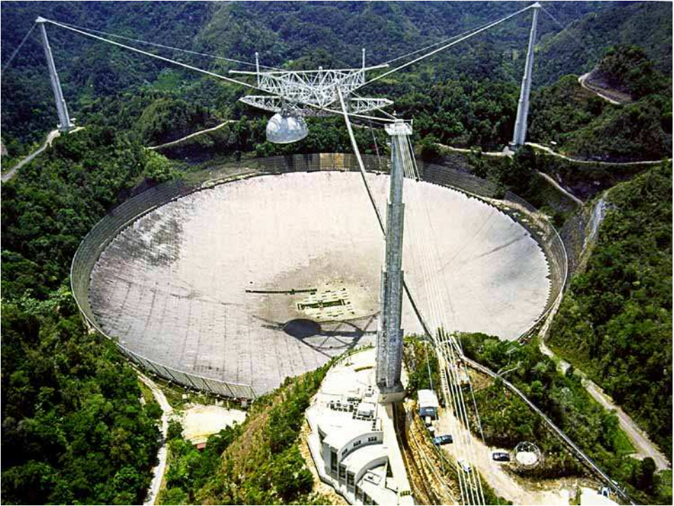
Fig. 11.1 The Arecibo radio antenna (telescope) consists of a 1000-foot fixed reflecting surface, made up of 40,000 individual panels, suspended in a natural limestone sinkhole in northwestern Puerto Rico. Incoming rays are reflected back from the surface to two additional reflectors located 450 feet above on the “platform”, a 500-ton structure supported by cables from three towers. Credit: NAIC and NSF.
