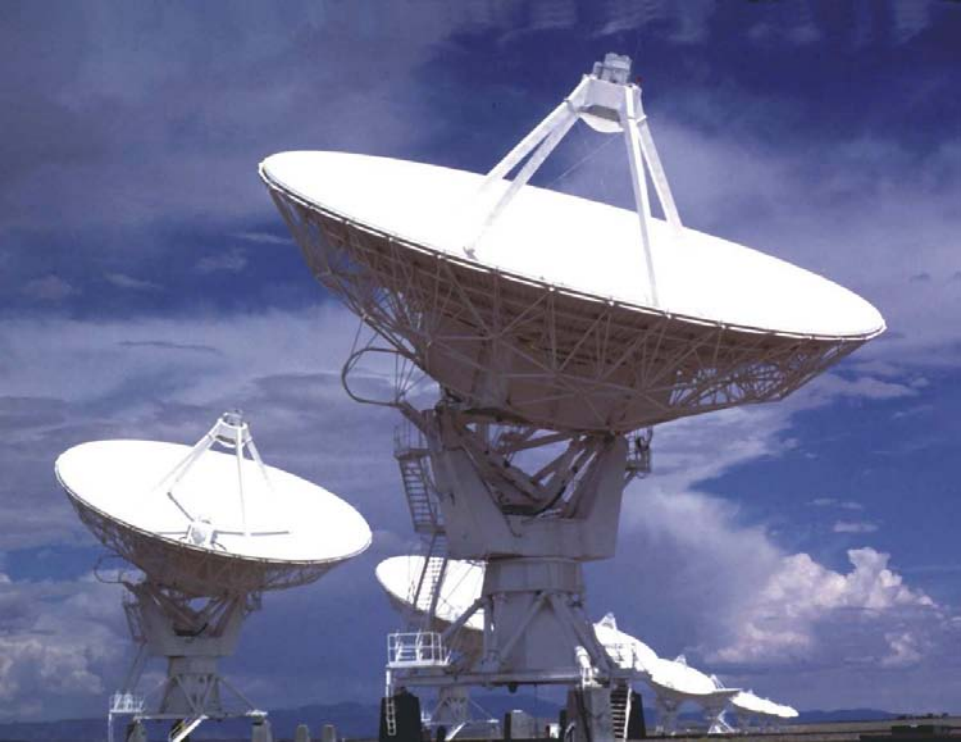
Fig. 4.12 A view of part of the Very Large Array in New Mexico. These “dishes” are antennae, tuned to detect the long-wavelength radio waves from pulsars. Credit: NRAO/AUI/NSF.
