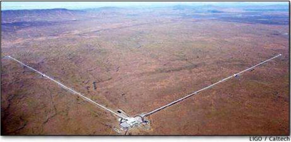
Fig. 8.6 An aerial photograph provides a sense of the massive scale of the Laser Interferometer Gravitational-Wave Observatory on the Hanford Nuclear Reservation. Eventually, the L-shaped facility will stretch 2.5 miles (4 km) in each direction.
