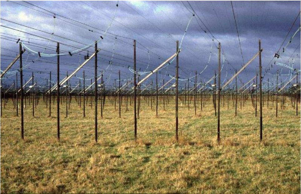
Fig. 4.7 The 4-acre antennae array of Hewish and Bell, from which the first pulsar signals were discovered in 1967 at Cambridge University. The discovery was serendipitous — pulsars (neutron stars) had not previously been known to exist. Compare this with a modern antenna in Figure 4.12.
