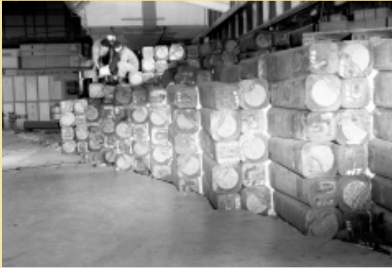
Building the shielding for the CERN neutrino experiment.
