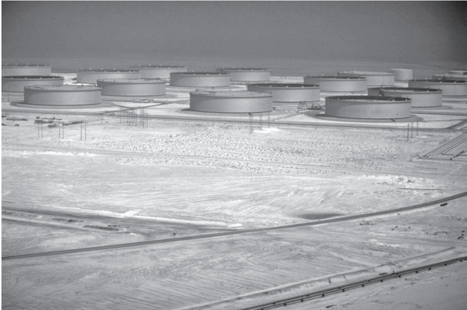
Petroleum tanks in Dhahran, Saudi Arabia. (Corel)
