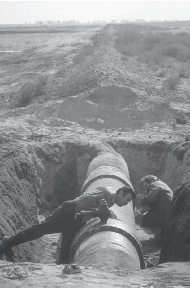
Workers inspect an oil pipeline in Saudi Arabia. (Saudi Aramco World/SAWDIA)
