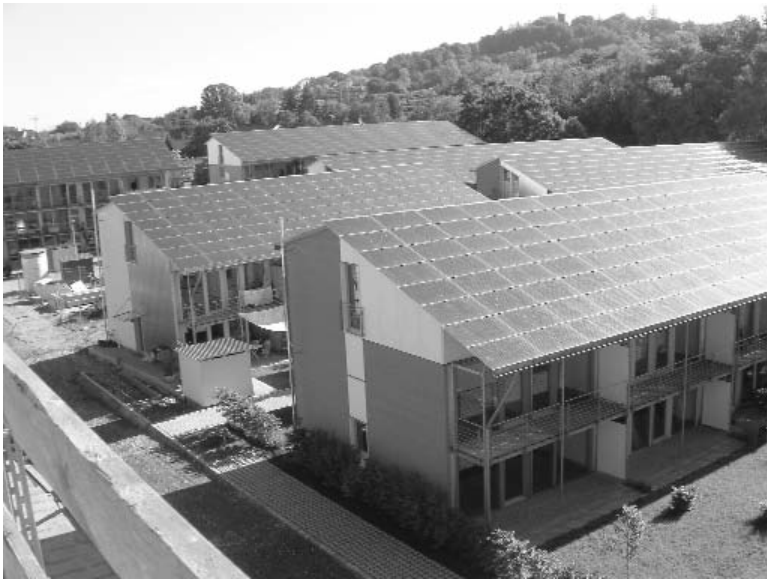
Vauban is a car-free eco-village that is setting new standards for sustainable urbanism and solar power. Shown above are the plus-energy homes that produce more energy than they need. (Credit: CABE/Alex Ely)
