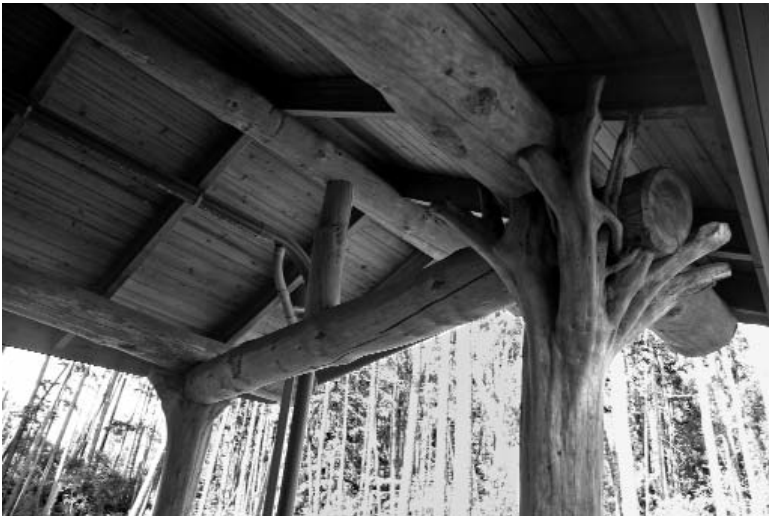
Astoria Bank building in Oregon demonstrates localism and green features. (Credit: Timothy Beatley)
