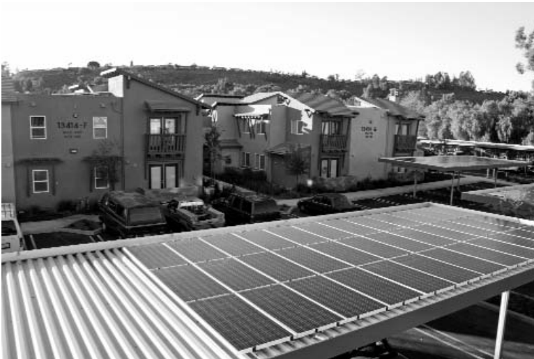
Green buildings provide the basis for carbon neutral cities. (top) CH2 building for Melbourne City Council (Credit: City of Melbourne); (bottom) Solara in San Diego (Credit: Timothy Beatley)
