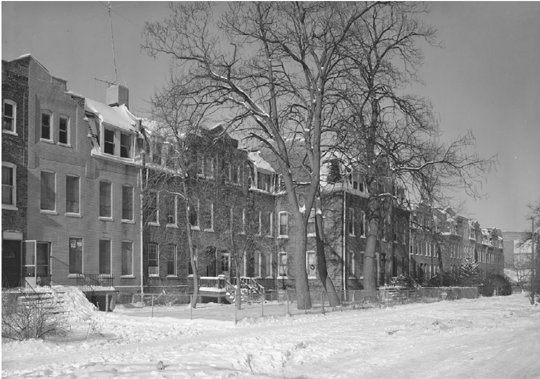
The company town of Pullman, Illinois, captured an idealized vision of industrial workers linked seamlessly as a unified work force. Workers' houses in Pullman, photographed here in the late twentieth century, provided shelter but also provided the means for the company to exert further control over its labor force. (Historic American Buildings Survey/Library of Congress)
