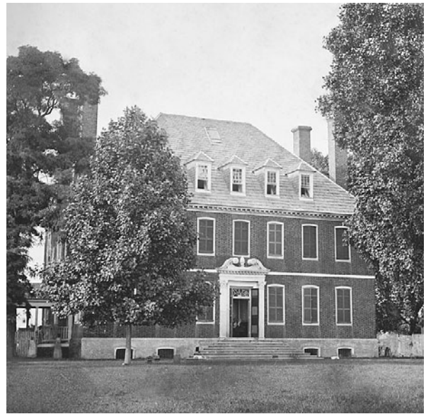
Westover, the house built by planter William Byrd II in the mid-eighteenth century, commands a view of Virginia's James River. The brick building's symmetry, entranceway pediment, and hipped roof are features of the Georgian style. (Library of Congress)
