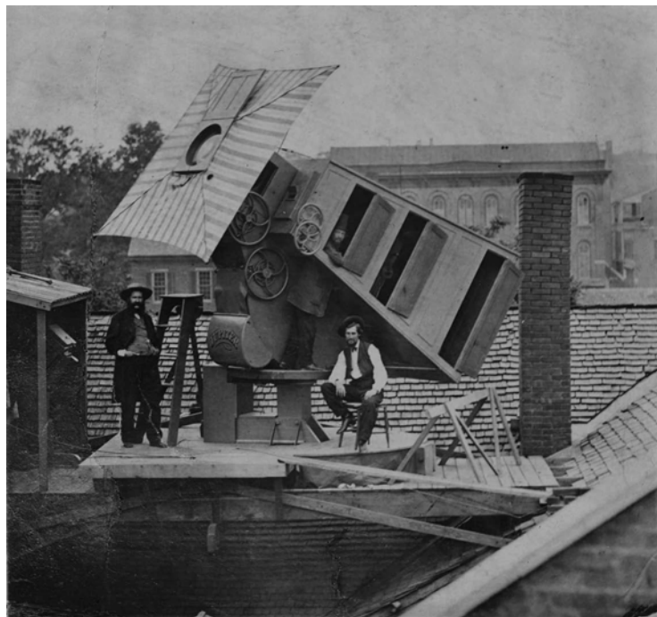
The Jupiter enlargement machine on the roof of Van Stravoren's studio, 1866. Barnard's first duties were to maintain the alignment of the aperture with the Sun. J. H. Van Stravoren is on the left, J. W. Braid inside the camera, and an unidentified man is seated.
