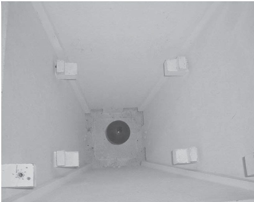
Figure 6-5: Exposure cone cleat placement
