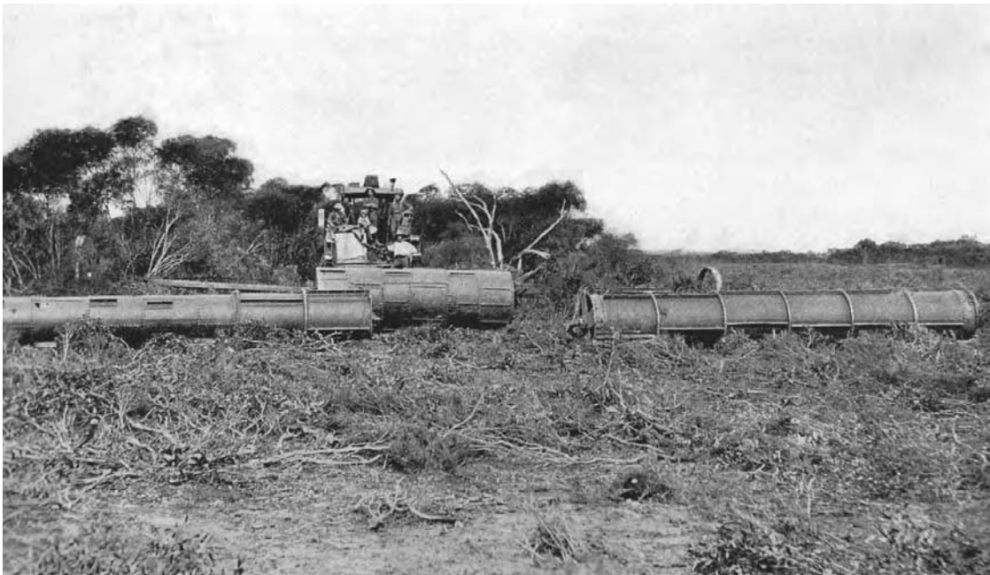
Mallee lands were easier to clear than forests and various methods were developed, such as dragging huge rollers through the bush. The broken trees could then be gathered and burned. (E. J. Brady, Australia Unlimited , Melbourne, 1918, p. 337)
