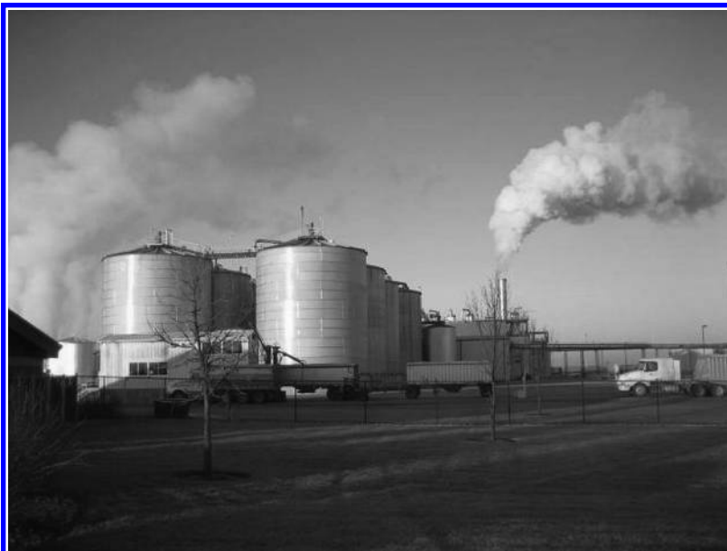
FIGURE 5.9 Fermentation tanks at a 120 million gal/y (450 million L/y) plant (author's photograph).
