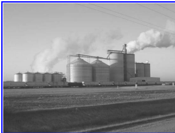
FIGURE 2.4 A typical dry grind corn-to-ethanol manufacturing plant. This plant has a nominal production capacity of approximately 120 million gal/y (450 million L/y) (author's photograph).
