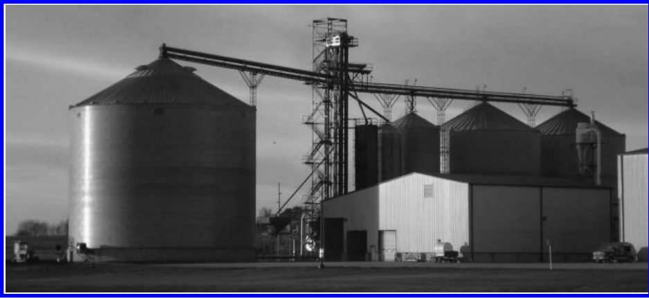
FIGURE 5.4 Corn is conveyed vertically by bucket elevators, and horizontally by drag conveyors. Note the drag scalper between the bucket elevator discharge and the distribution conveyor—it is used to clean the incoming grain. This is a 21-million gal/y plant (author's photograph).
