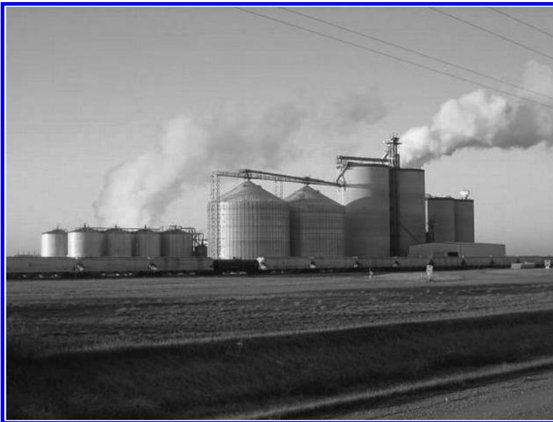
FIGURE 5.5 A large-scale ethanol plant often uses both types of grain storage options. Large concrete silos are generally constructed with the original facility, and steel bins are then installed during future expansions. Note the small concrete silos used for DDGS storage. This is a 120-million gal/y (450 million L/y) plant (author's photograph).
