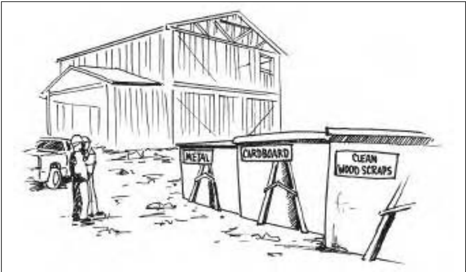
FIGURE 11.4— Sorting waste materials into different bins will make delivery of those materials to the recycling facility (or facilities) easier and also keep the job site tidier.
