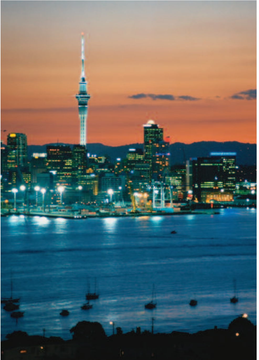
The Sky Tower in the city of Auckland is the highest structure in the Southern Hemisphere.
