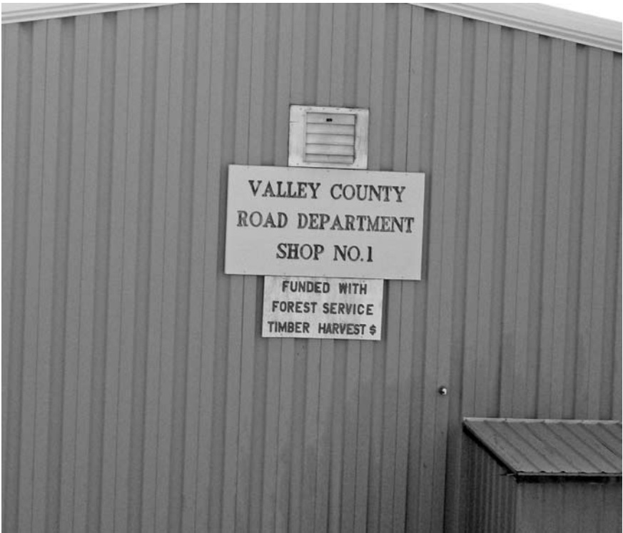
Photo 1.1 Valley County Road Department Shop No. 1. Funded with Forest Service Timber Harvest $.
