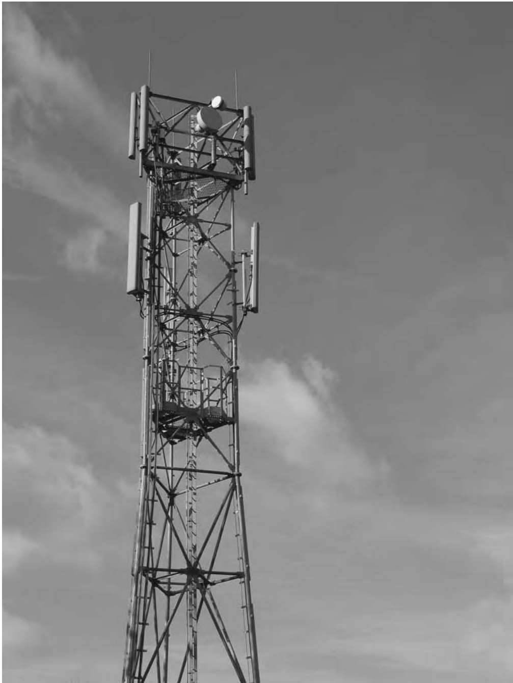
Figure 4.7 A typical cellular telecommunications base station with its antenna tower.
