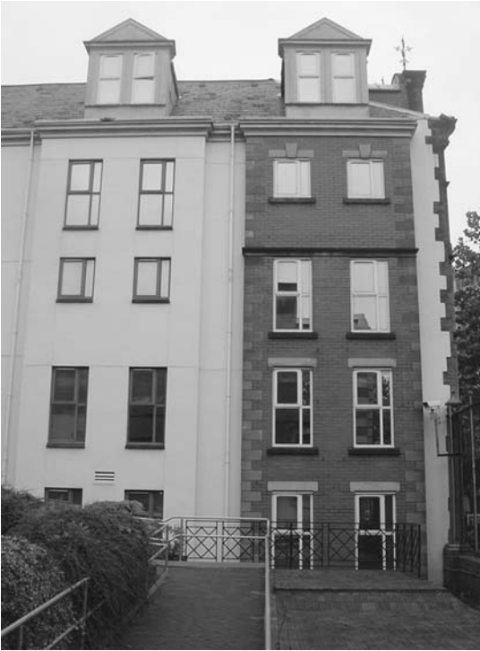
▲ E6 The successful marrying of old and new on south-west façade
