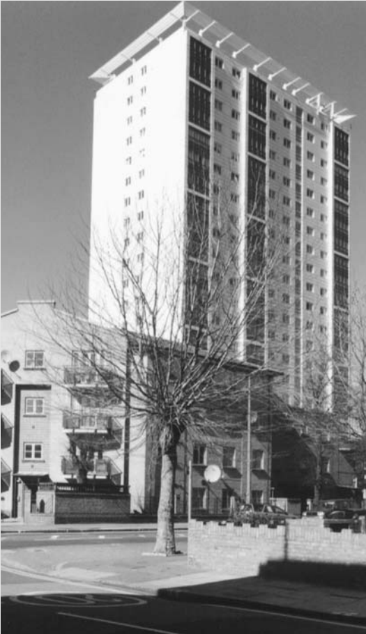
▲ 6.5 The improved tower block reserved for older residents
