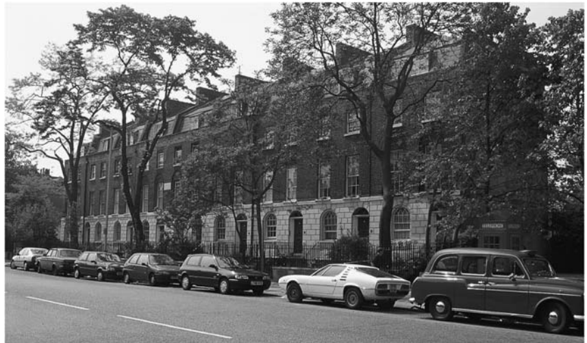
▲ 0.8 Old terraced housing renovated and converted
