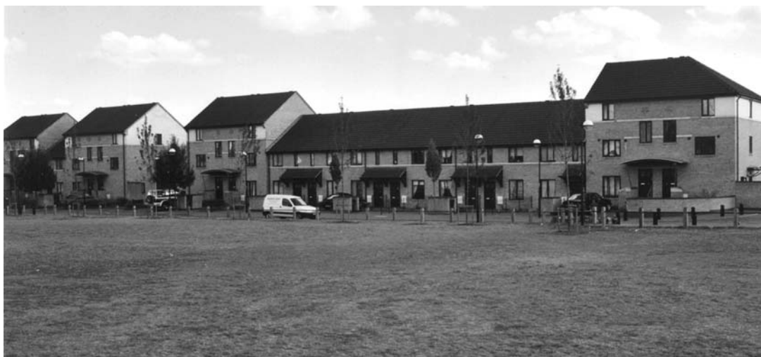
▲ C4 Social housing around the new 'village green'
