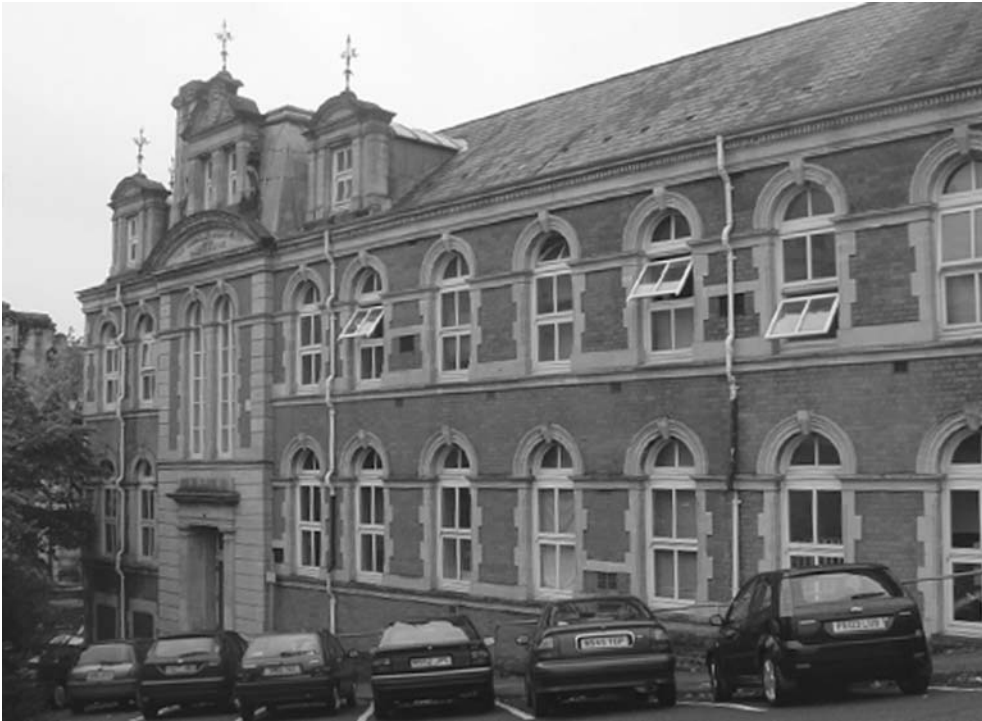
▲ E2 The Retained north-east façade which marries with new structure behind
