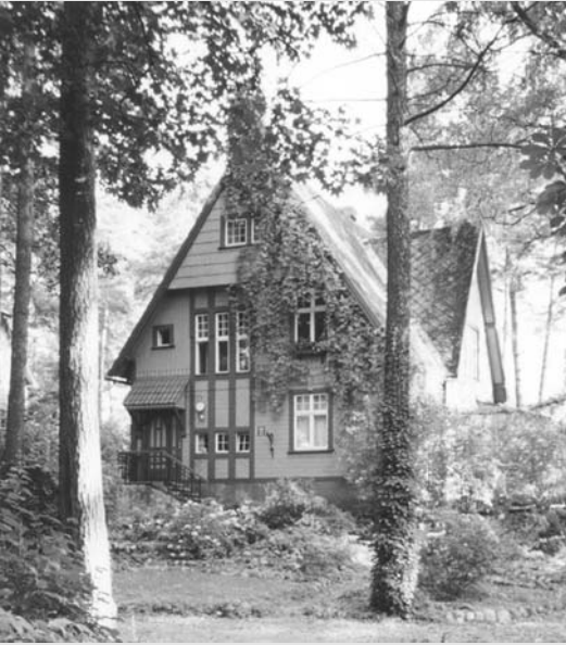
▲ 8.7 House in the resort of Jurmala
