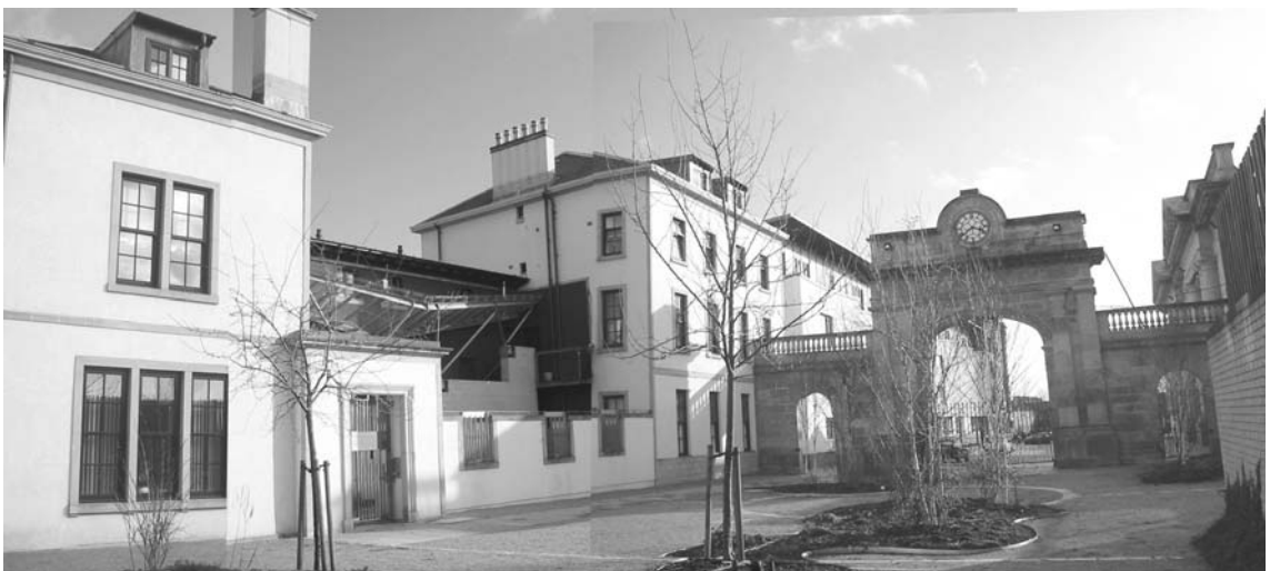
▲ 6.8 Conversion of a listed hotel to flats – Part of a complex of new housing at Graham Square Glasgow. A two-storey infill block has been built between the two existing buildings to provide more accommodation and a new main entrance
