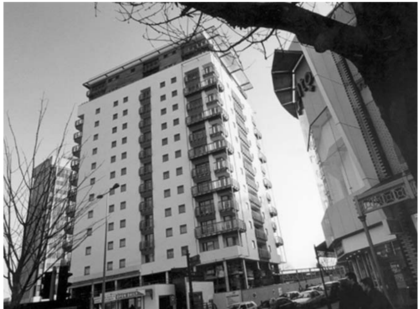
▲ 6.7 The Aspect Cardiff – former offices of the AA Insurance Service converted into flats. The project was completed in 2002 and comprises 99 one, two and three-bedroom apartments. Two new floors have been added to provide penthouse maisonettes
