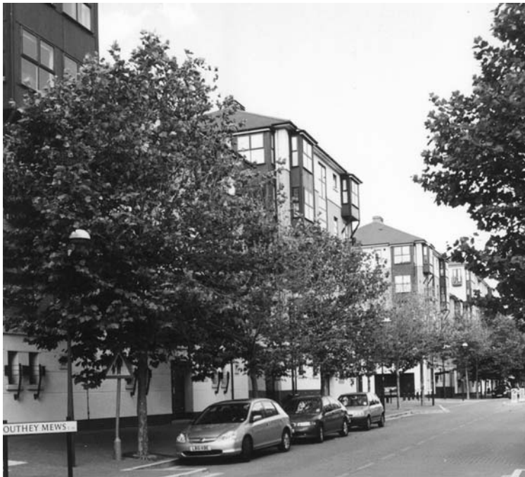
▲ C6 Six-storey blocks along the central road
