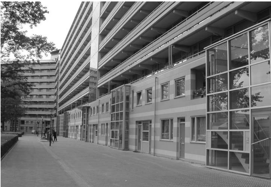
▲ K2 New maisonnettes and entrances built into lower levels of multi-storey block
