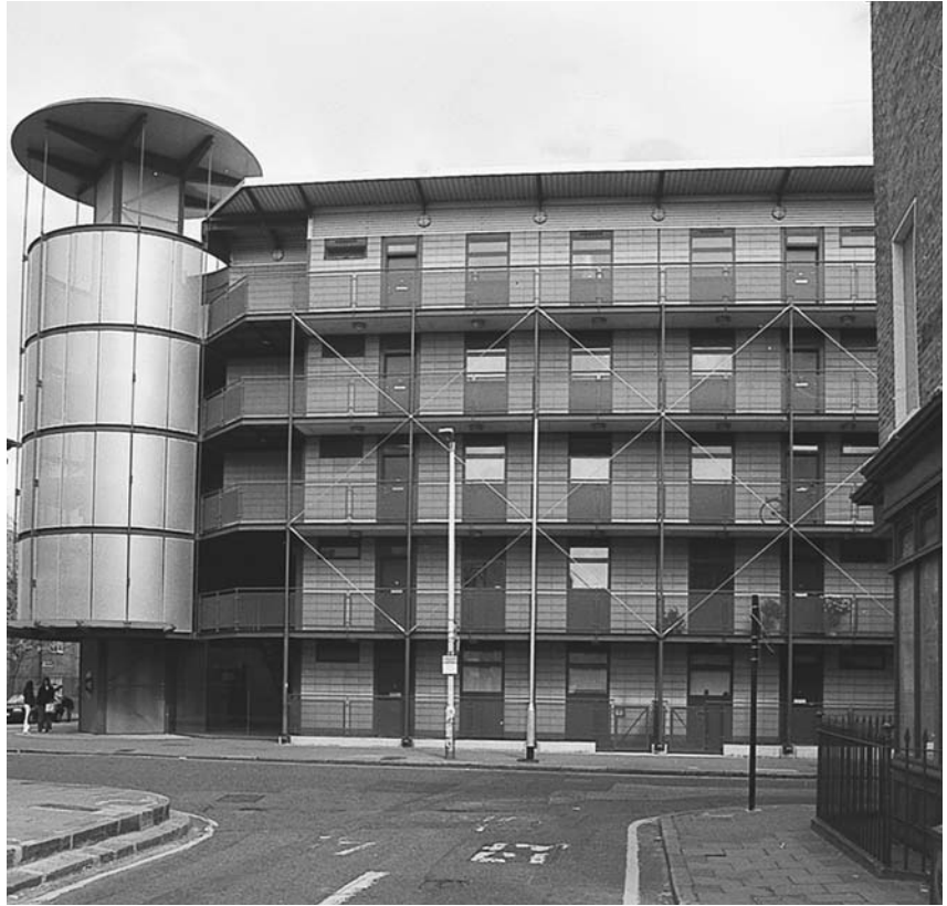
▲ 5.5 Murray Grove, pioneering project using modular construction
