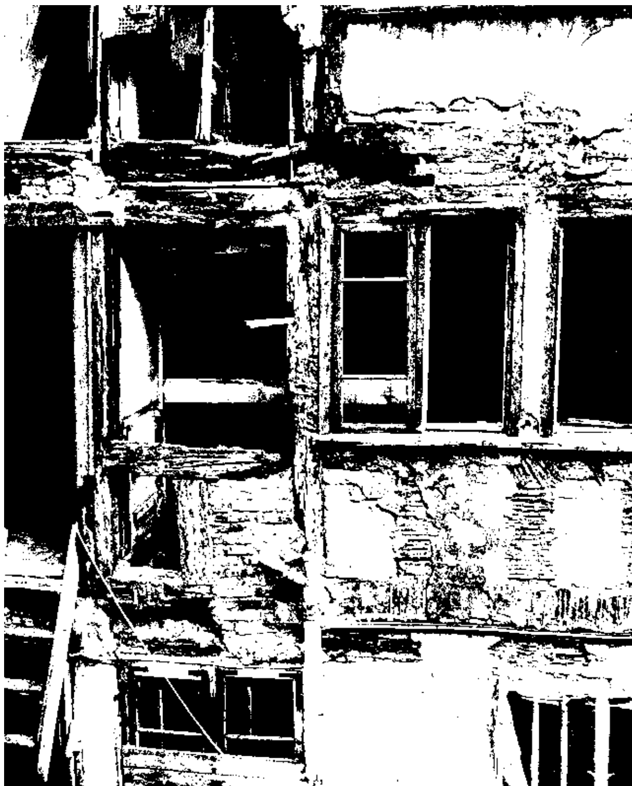
Figure 4.9 One of the three houses at Christianshaven, Copenhagen, Denmark (Courtesy: Architects W. Wohlert and H. Laugberg and J. Fredstund)
