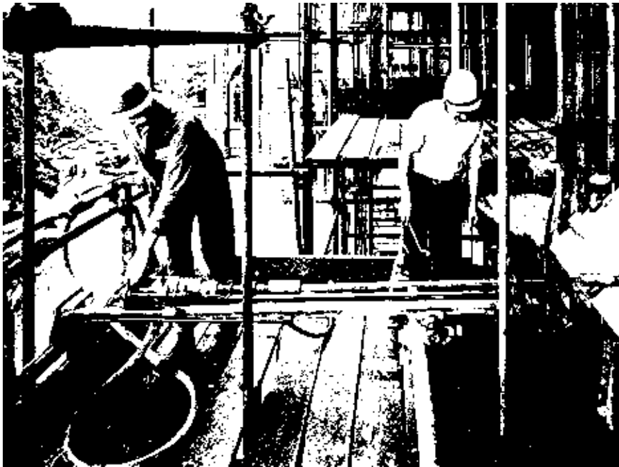
Figure 21.19 Drilling, York Minster, England (Courtesy: Shepherd Building Group Ltd)
