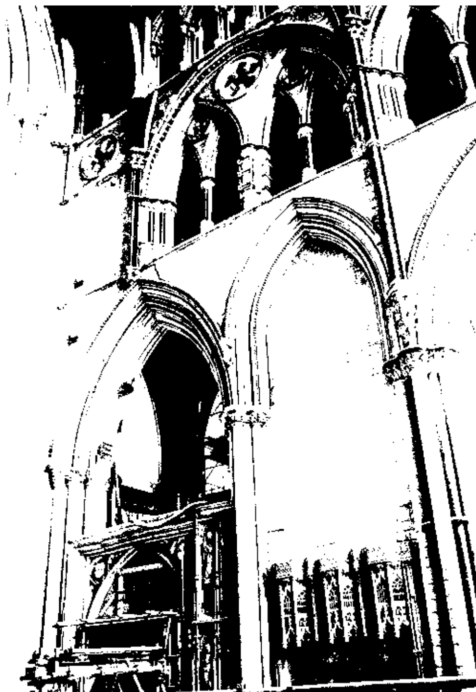
Figure 14.3 South transept, east arcade, and tower abutment, York Minster, England
