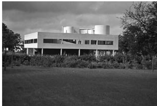
Figure 22.1 Villa Savoie, Poissy, Paris, 1930 (Photograph: John Allan, Avanti Architects, London)
