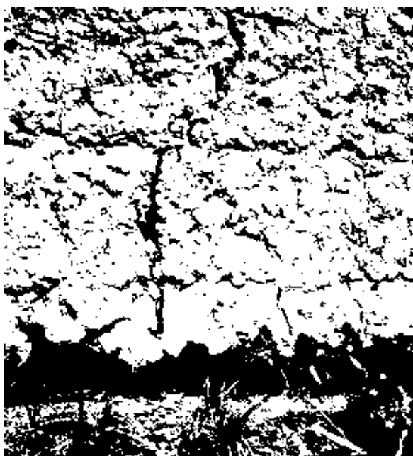
Figure 5.7 Modern mud wall near Kerbala, Iraq
