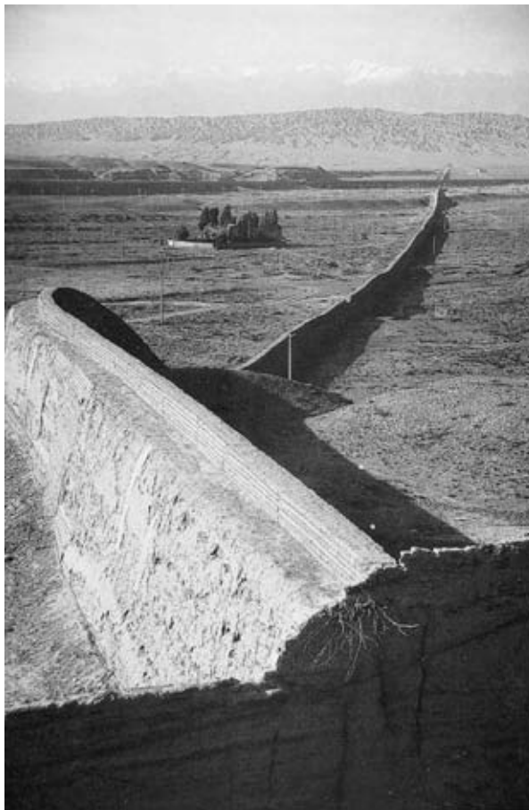
Figure 5.9 The Great Wall of China—the western end at Giau Guan. Famed as man's largest historic construction, the Wall is an earth structure throughout its length, although stone-faced at its eastern end (Courtesy John Warren)
