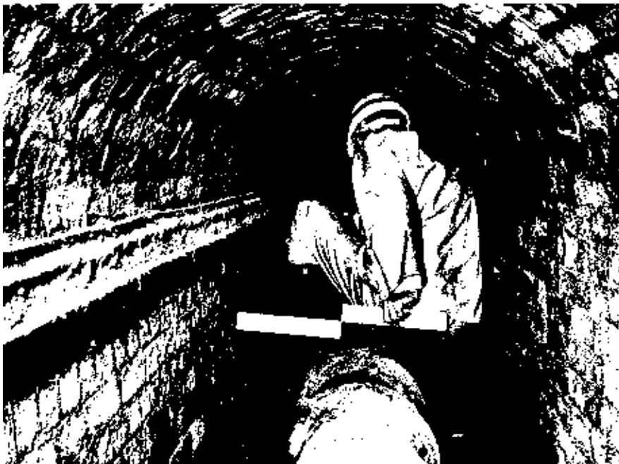
Figure 14.11 Original rainwater disposal system, St Paul's Cathedral, London, England
