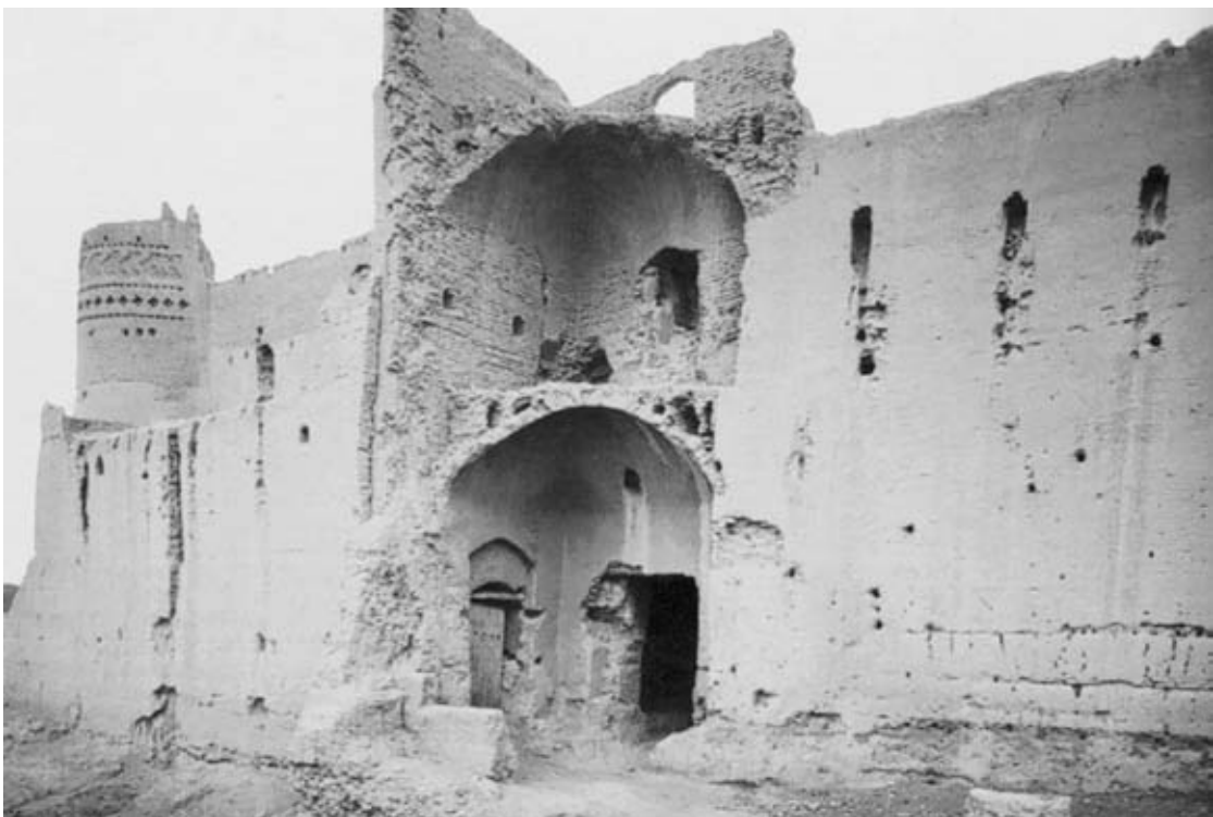
Figure 5.12 Iran: medieval castle at Faraj. The collapse of a double-chambered tower demonstrates the slender cross-sections achievable with the use of squinches and secondary vaulting in the haunches of vaults. These techniques are apparent from the early Middle Ages and precede the structural magic of Persian brickwork (Courtesy John Warren)
