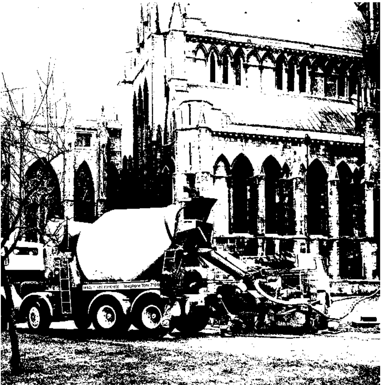
Figure 21.38 Pumping concrete, York Minster, England (Courtesy: Shepherd Building Group Ltd)
