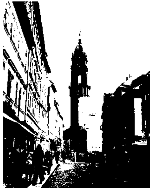
Figure 6.12 Tower, Bautzen, Germany (Courtesy: Ing. W. Preiss)
