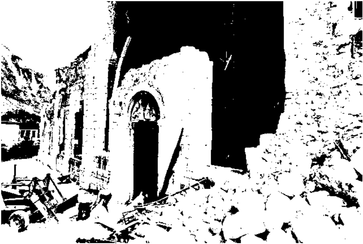
Figure 8.4 Friuli, Italy (Courtesy: Architect G. Tampone) Earthquake damage
