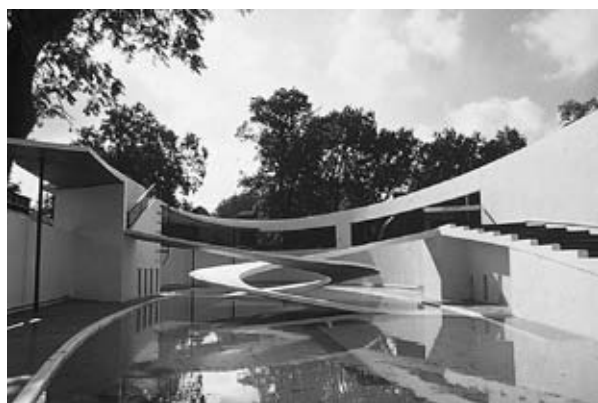
Figure 22.2 The Penguin Pool, London Zoo, England, 1934 (Photograph: John Allan, Avanti Architects, London)
