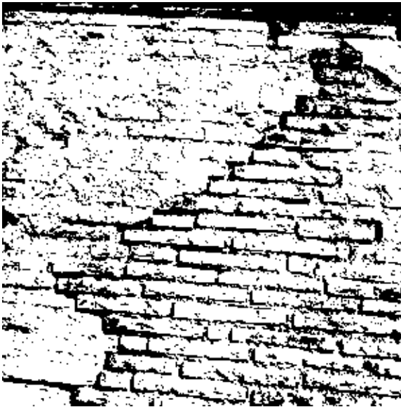
Figure 18.7 The Pantheon, Rome, Italy (detail of brickwork on the drum)
