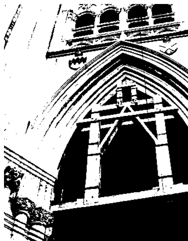
Figure 21.3 Shoring, choir, north arcade, York Minster, England
