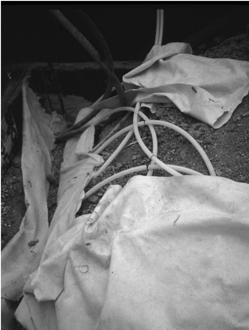
Figure 7.7 Photograph showing installation of ground coils.
