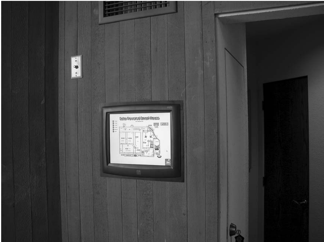
Figure 7.10 Photograph showing color touch screen wall mount.
