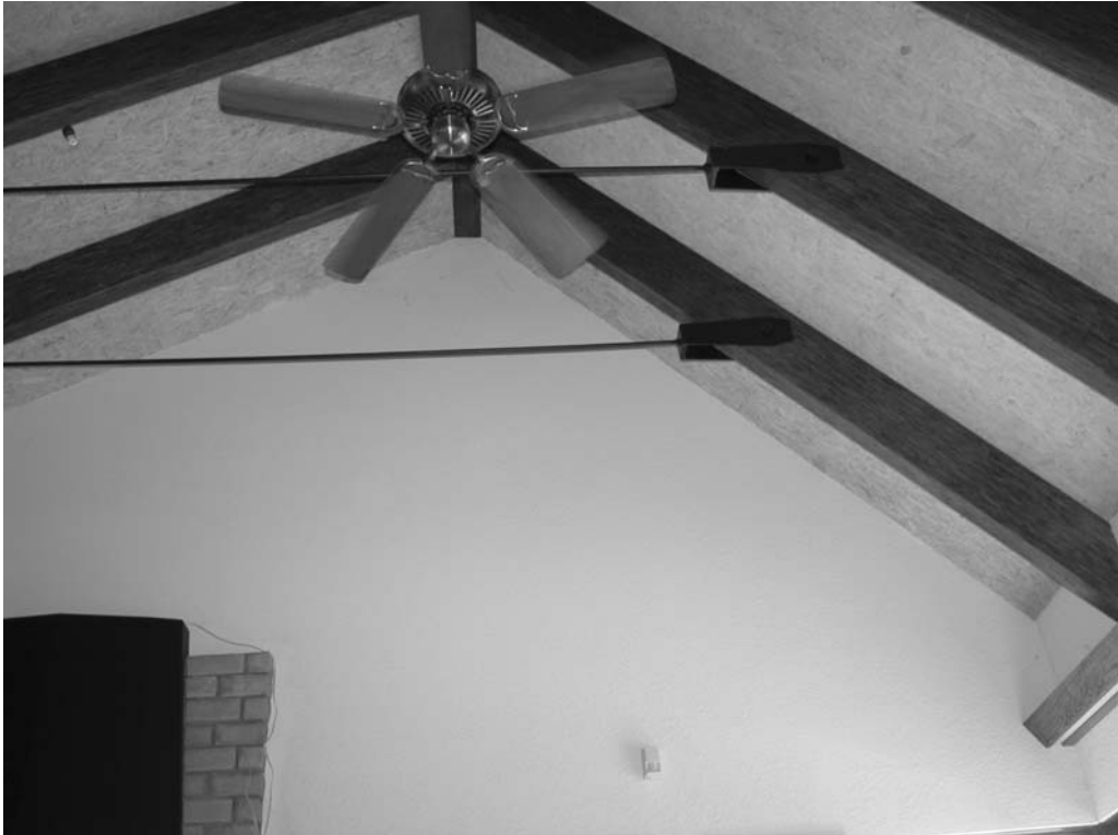
Figure 7.3 Exposed beam ceiling inside of 45° slope roof.
